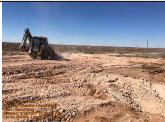
Backfilling
