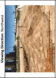
2 ft excavation area going back towards pad area where 0.5 inch excavation occurred
