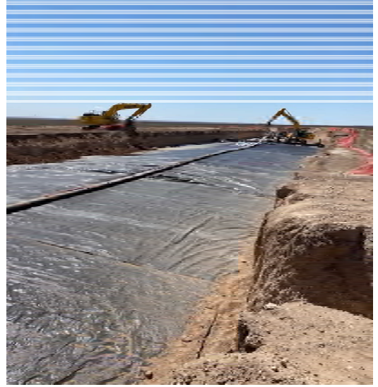
Liner Installation Midway-Complete
