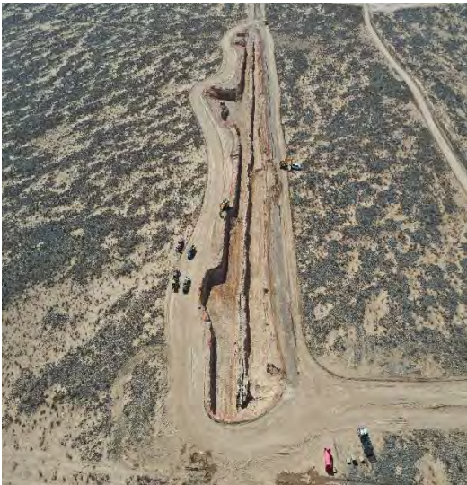
Aerial of entire excavated area
