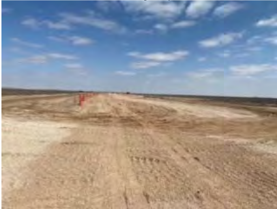
Backfilled to grade
