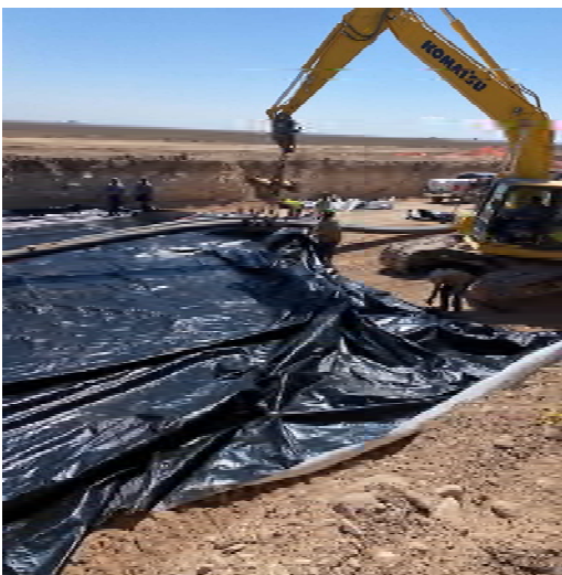
Liner install under lines
