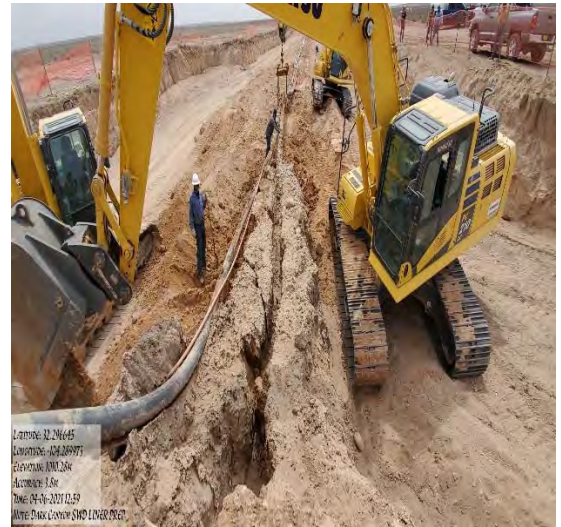
Preparation under lines for liner install
