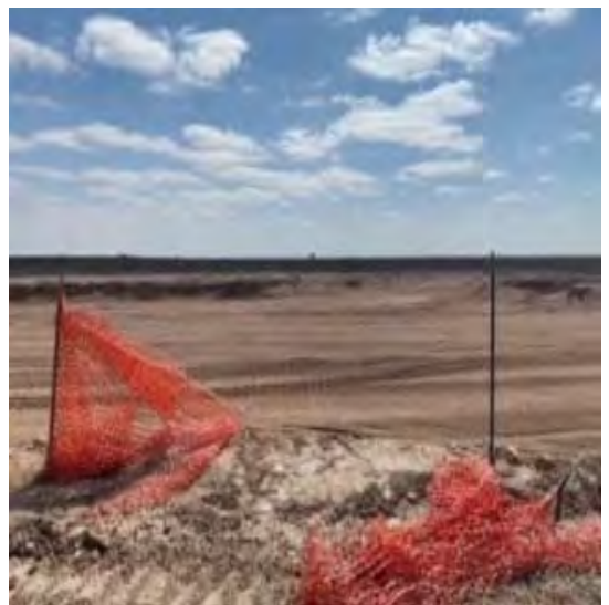
Backfill @ Center to grade
