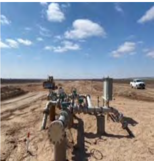
Backfill @ Source to grade
