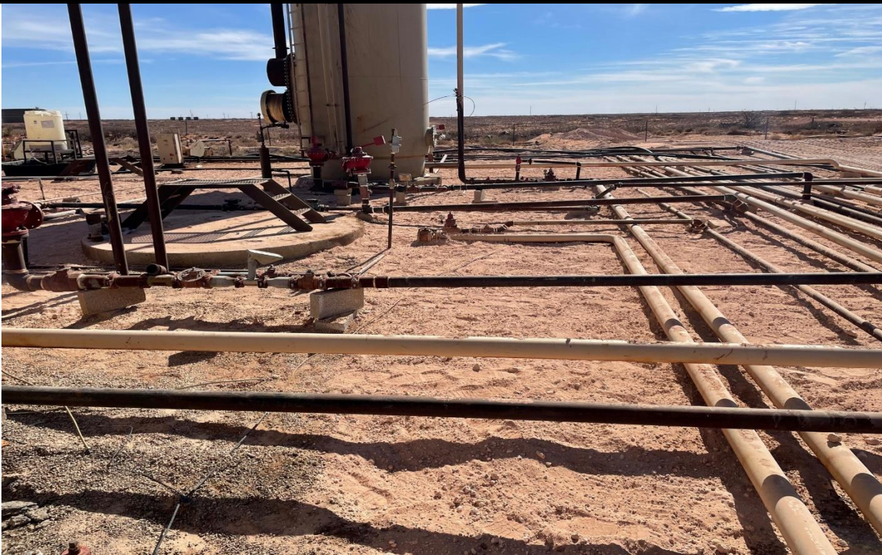
PHOTO 12: View of tank battery and remediated area, facing east. 2/3/2021
