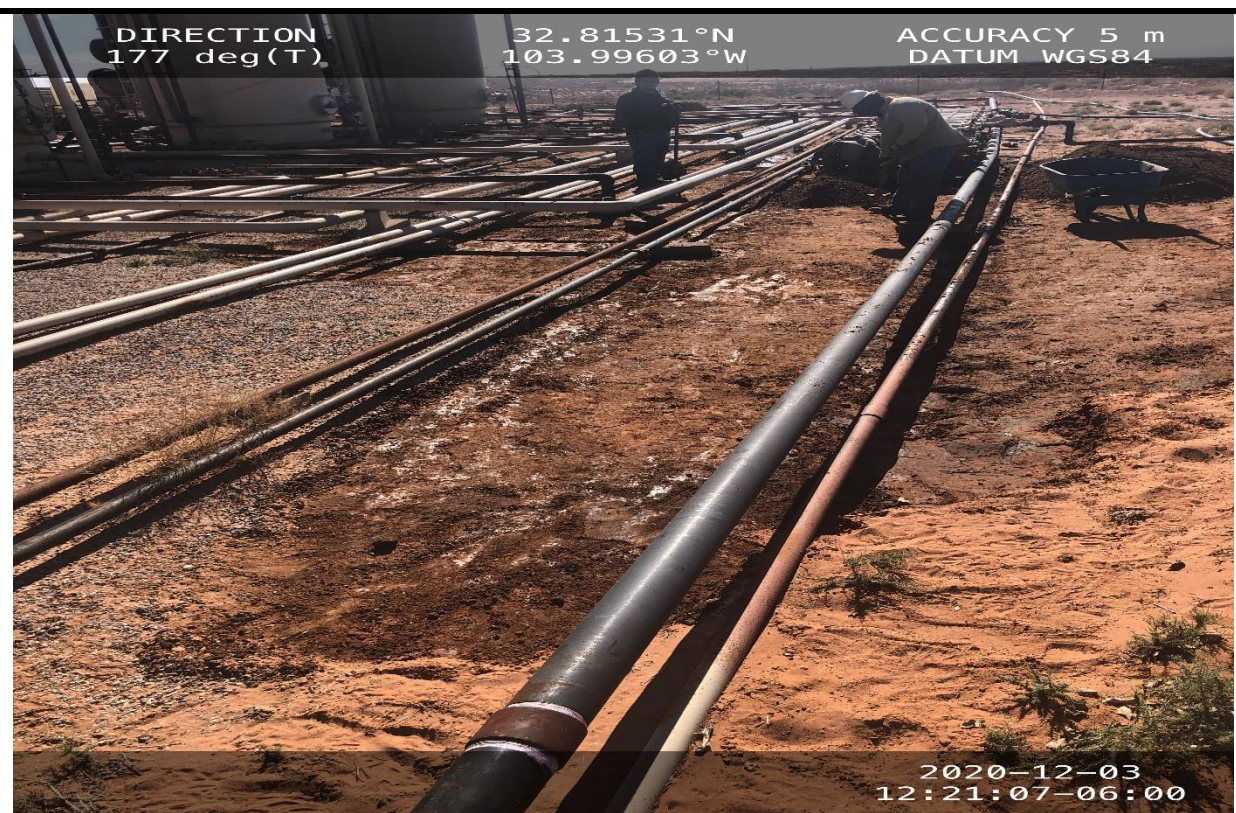
PHOTO 5: View of spill and tank battery, facing south. 12-3-2020
