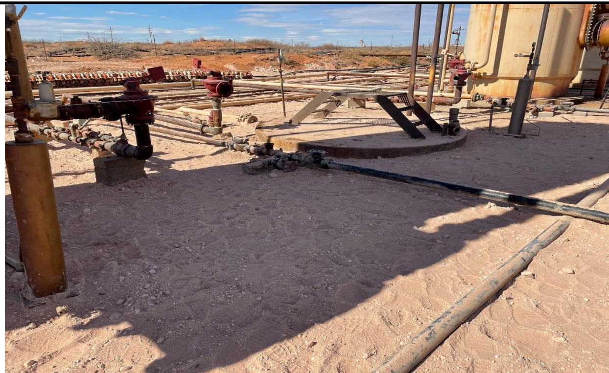
PHOTO 18: View of tank battery and remediated area, facing northwest. 2./3/2021
