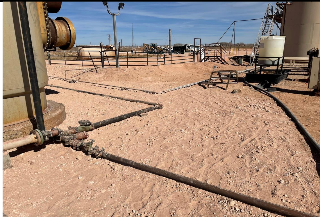
PHOTO 17: View of tank battery and remediated area, facing northeast
