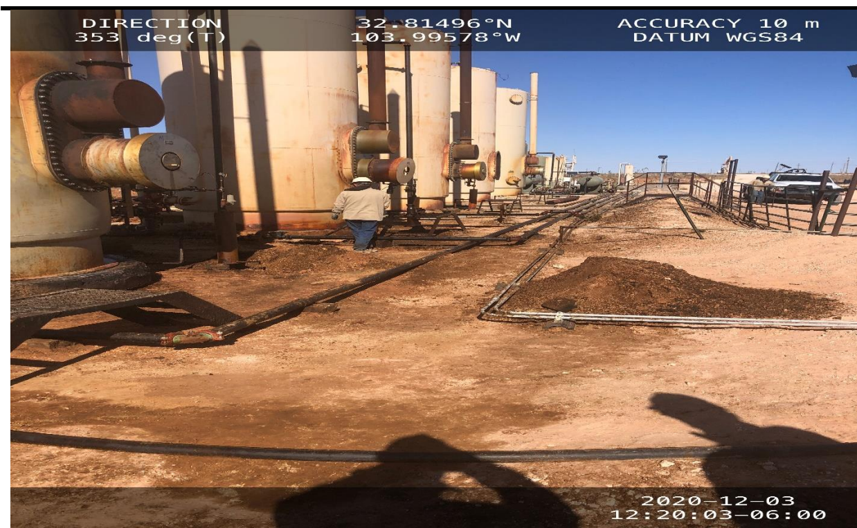
PHOTO 1: View of spill and tank battery, facing north. 12-3-2020
