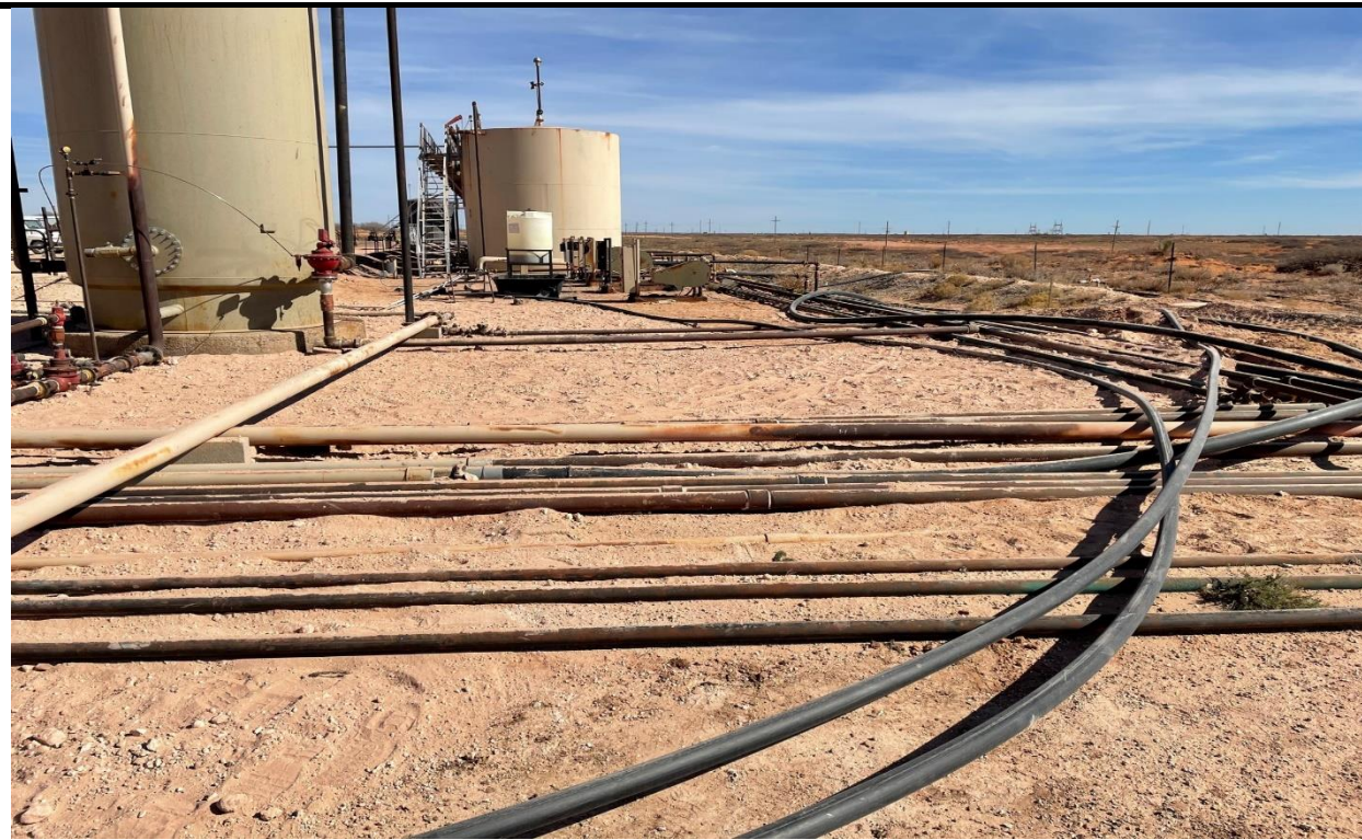
PHOTO 16: View of tank battery and remediated area, facing east. 2/3/2021
