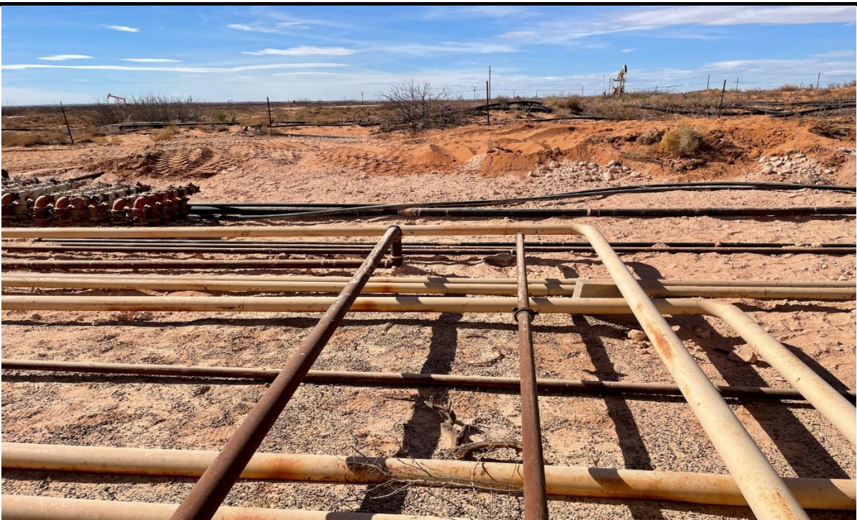
PHOTO 10: View of remediated area, facing west. 2/3/2021
