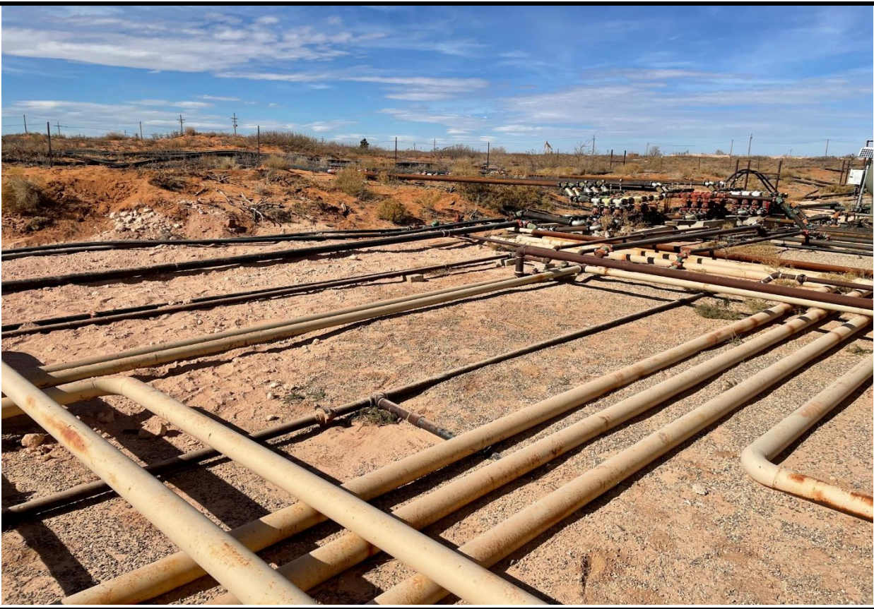
PHOTO 9: View of remediated area, facing northwest. 2/3/2021
