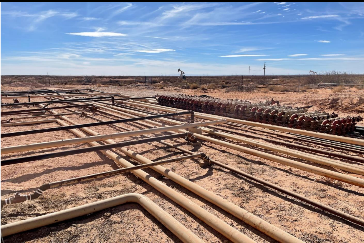
PHOTO 11: View of connectors and remediated area, facing southwest. 2/3/2021
