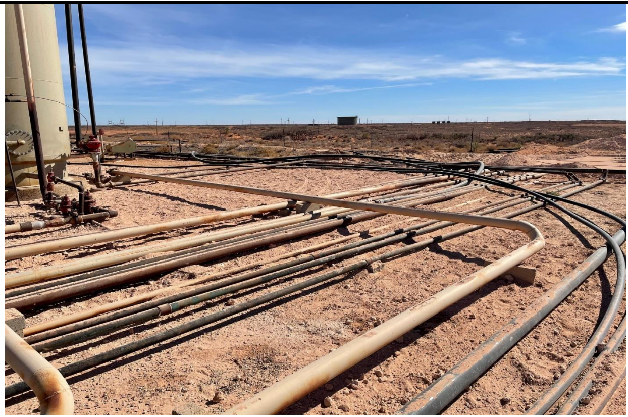
PHOTO 15: View of tank battery and remediated area, facing southeast. 2/3/2021
