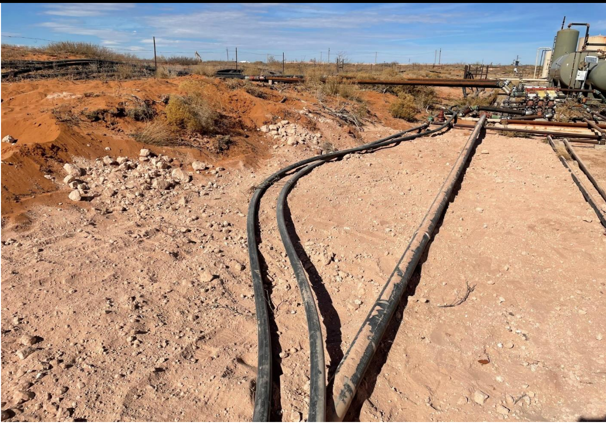
PHOTO 13: View of remediated area, facing north. 2/3/2021
