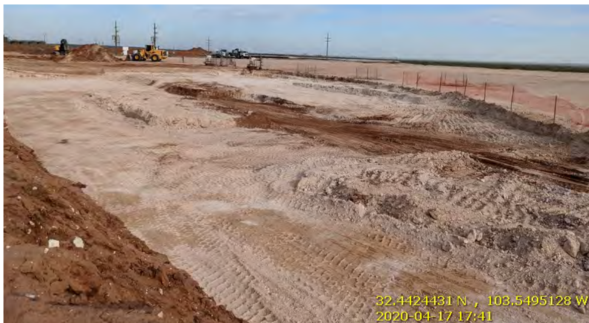
Photo 2: Photo viewing southeast from the north production pad wall. Excavation depth is an average 4.2-feet below production pad surface (8.2 feet below natural grade surface).
