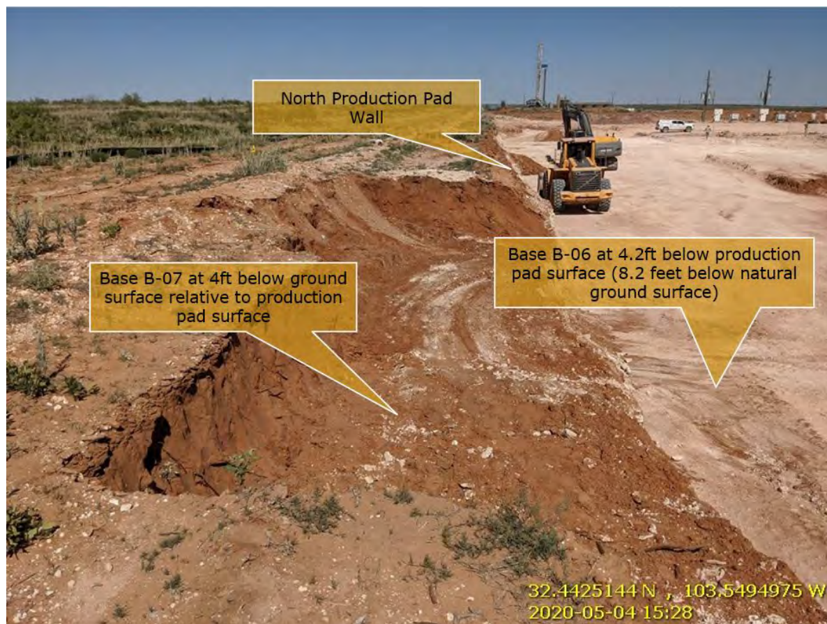
Photo 1: Photo viewing east along the north production pad wall. Area to the left (north) of the north production pad wall was remediate as off-site use along a pipeline right-of-way. The off-site area was excavated to a depth of 5-feet (or 1-foot below relative production pad surface).
