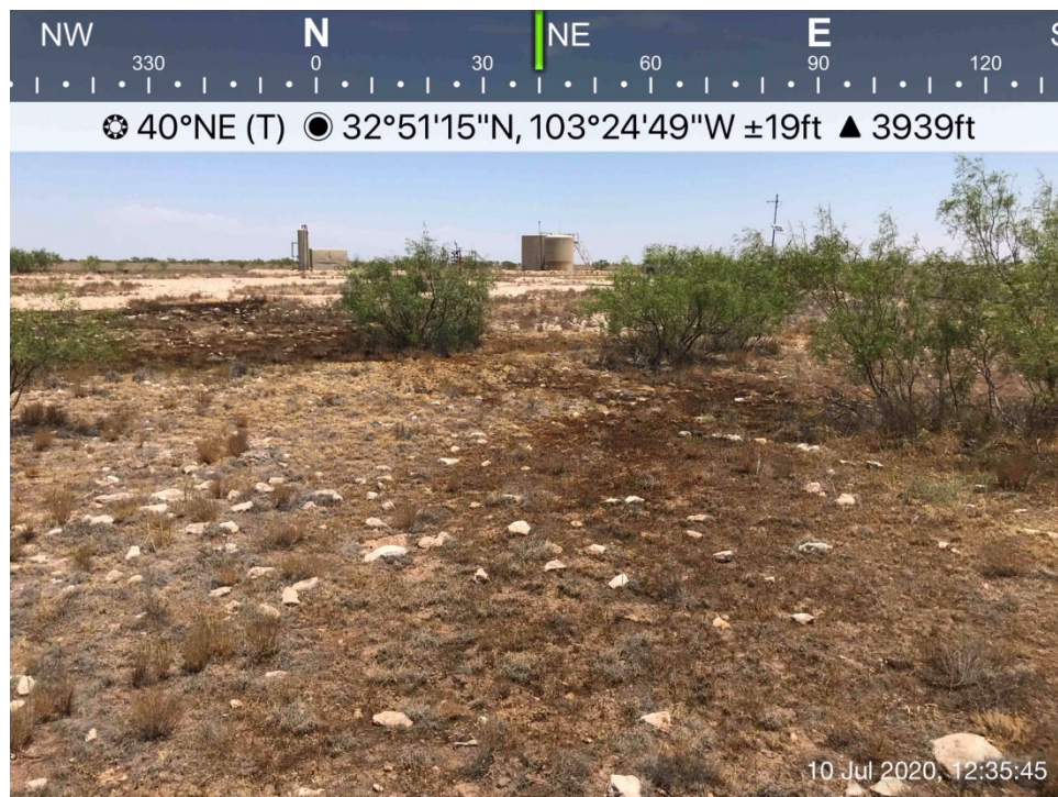
Impacted area viewing Northeast, July 10, 2020
