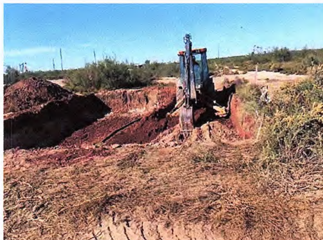
Excavating the site to 5 ft bgs, facing north
