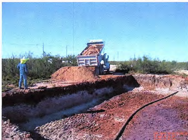
Excavation complete to a depth of 5-ft bgs and importing soil, facing northwest
