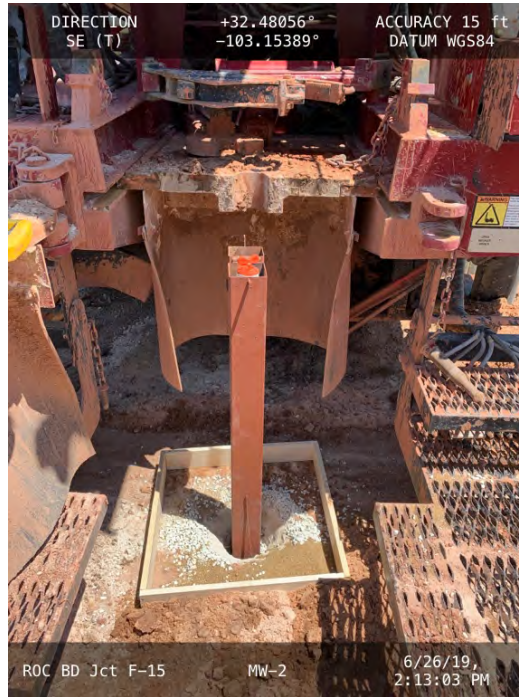
MW-2 Completion
