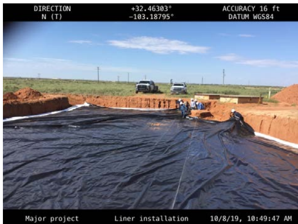
Installing and properly seating the 20-mil, reinforced liner, facing north 10/8/2019
