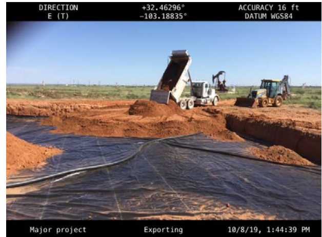
Backfilling and padding the liner with imported soil, facing east 10/8/2019
