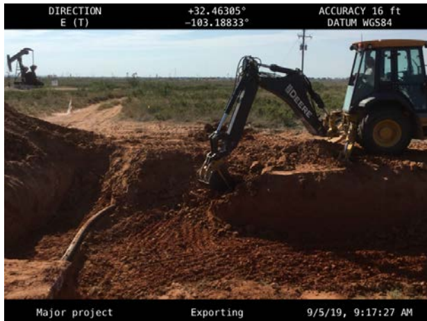
Excavating the site to a depth of 5 ft bgs, facing east 9/5/2019
