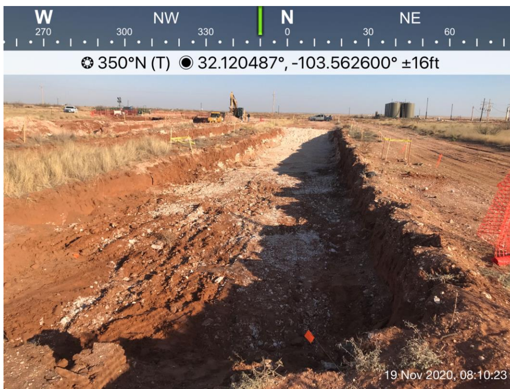
View North, area of Bottom Holes (81-92)
