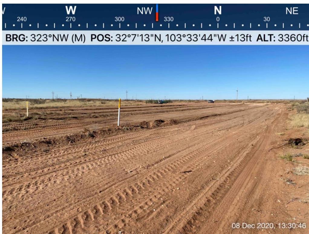
View Northwest, backfilled areas of Auger Holes (6-9)
