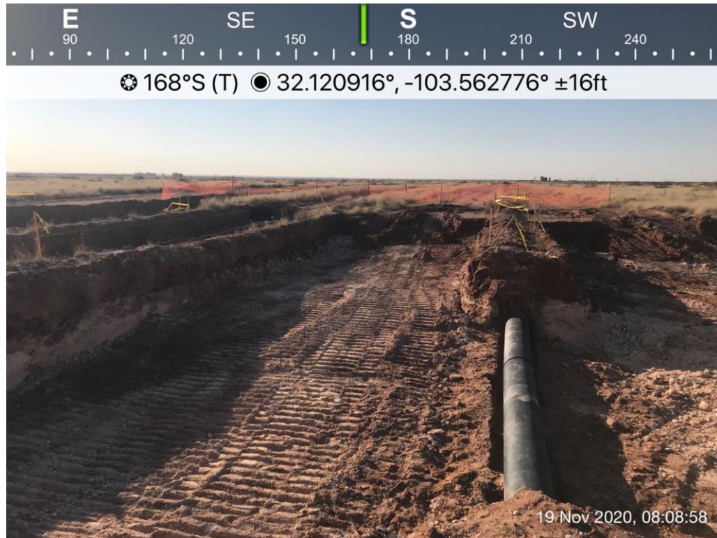
View South, area of Bottom Holes (11-20, & 51-61, & 93-94)
