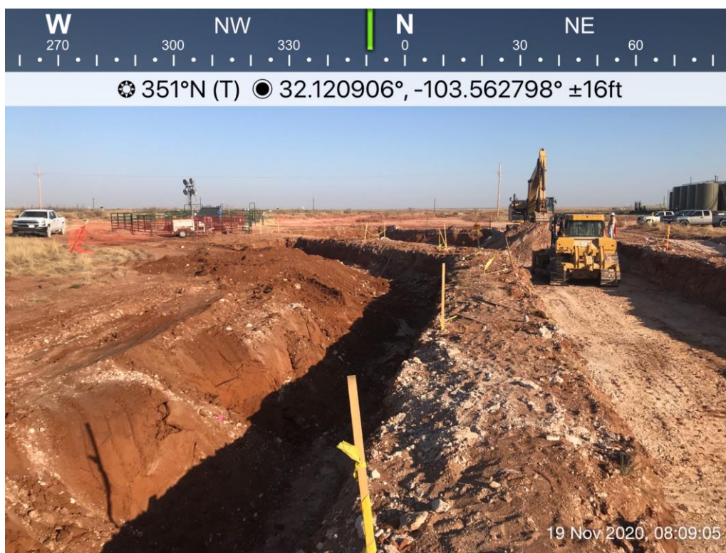
View North, area of Bottom Holes (1-10, & 21-50)
