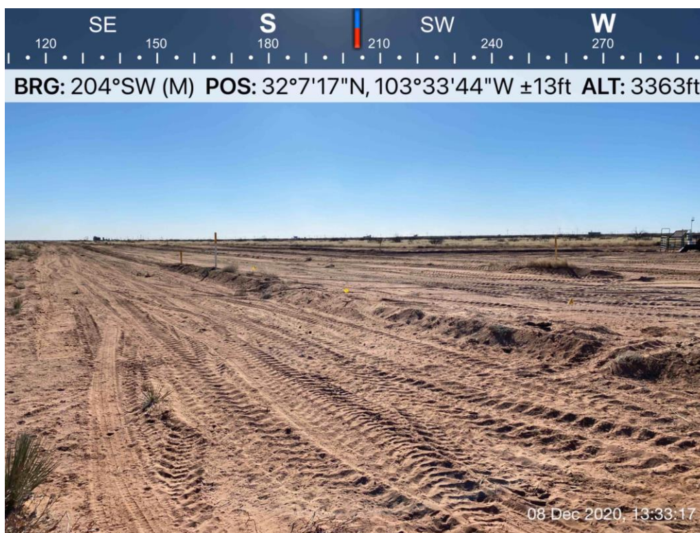
View Southwest, backfilled areas of Auger Holes (1-5)
