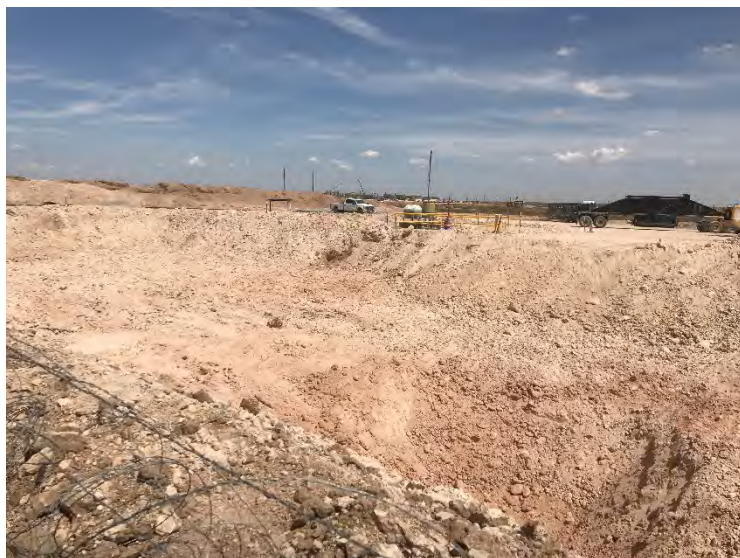
Photograph 9: View of open excavation on pad.
