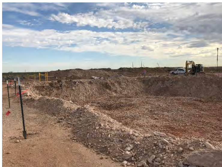
Photograph 7: View of open excavation on pad.
