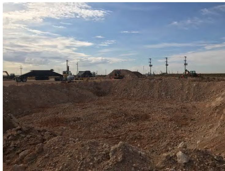
Photograph 6: View of open excavation on pad.
