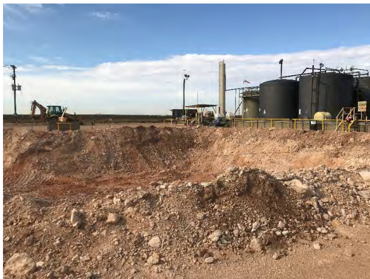
Photograph 5: View of open excavation on pad.
