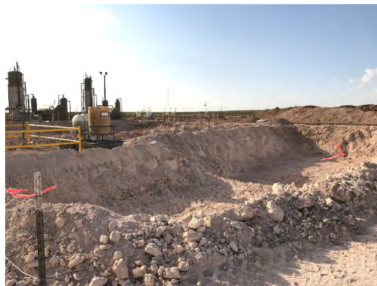
Photograph 8: View of open excavation on pad.
