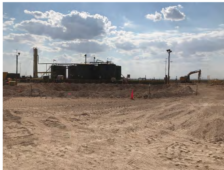
Photograph 10: View of open excavation on pad.
