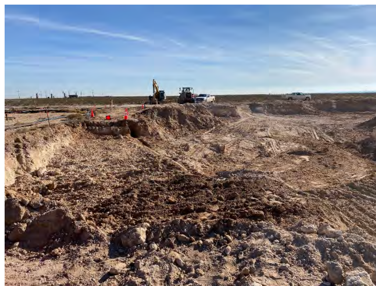
Photograph 16: View of open excavation in pasture.
