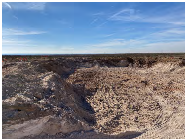
Photograph 15: View of open excavation in pasture.
