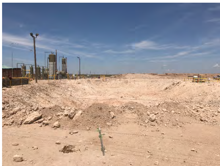
Photograph 11: View of open excavation on pad.
