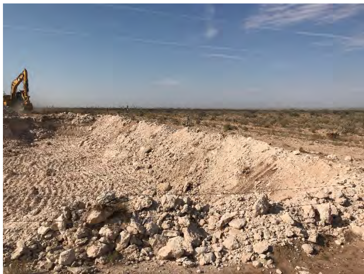
Photograph 13: View of open excavation in pasture.
