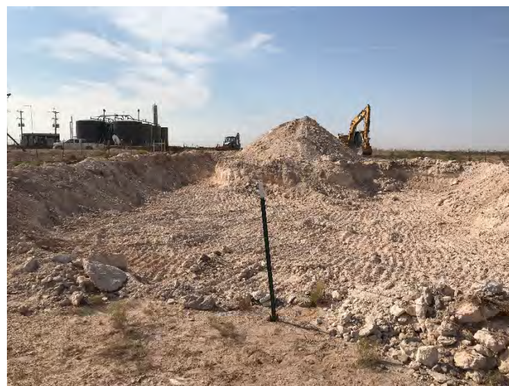
Photograph 12: View of open excavation in pasture.
