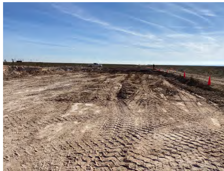
Photograph 14: View of open excavation.
