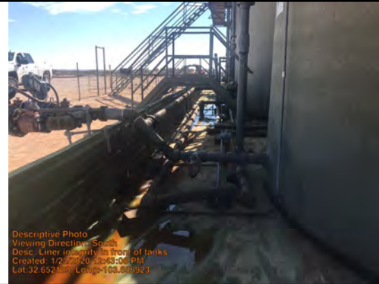
Liner integrity in front of tanks
