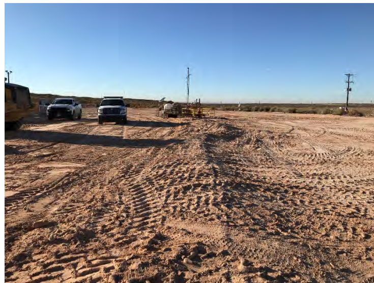
Photograph 10: West facing view after backfilling.
