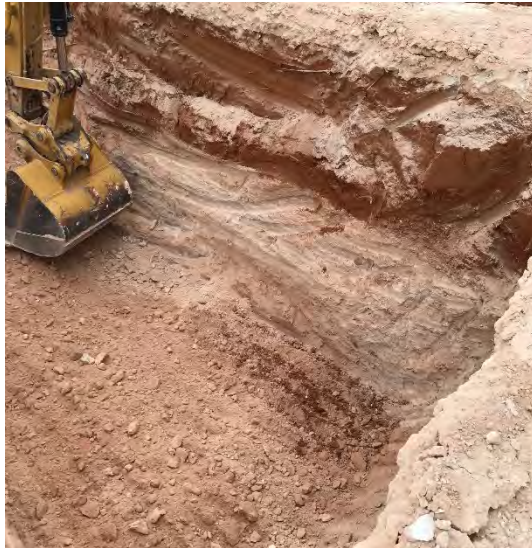
Photograph 3: View of open excavation near potholes PH02 and PH07.
