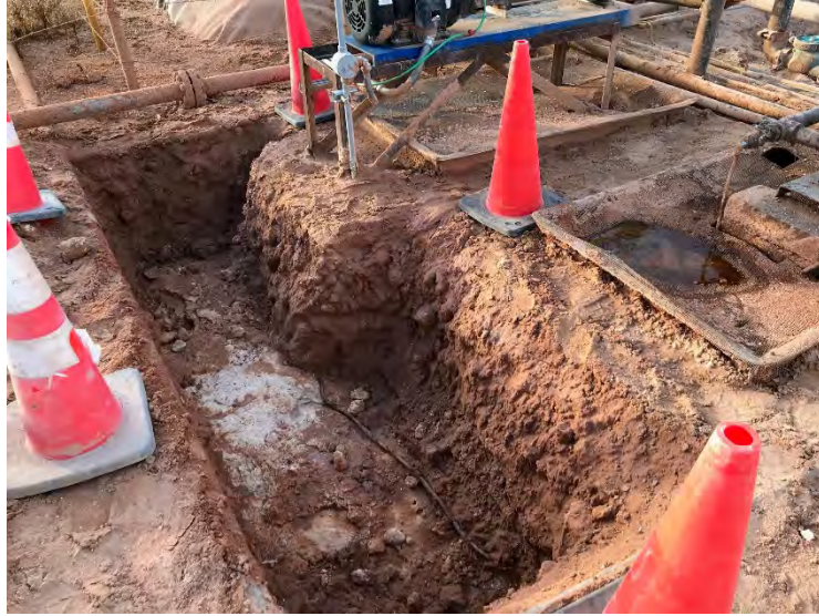
Photograph 1: View of hydrovac excavation and pipelines/equipment.
