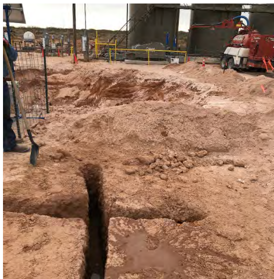
Photograph 5: South facing view during excavation activities.
