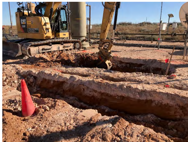
Photograph 6: Southeast facing view during excavation activities.
