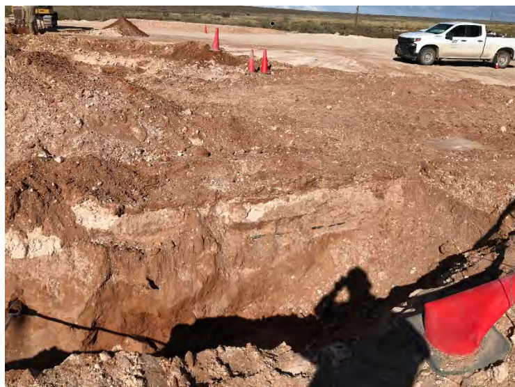
Photograph 7: View of open excavation near pothole PH01.
