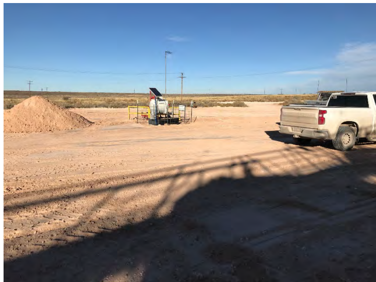
Photograph 9: North facing view after backfilling.
