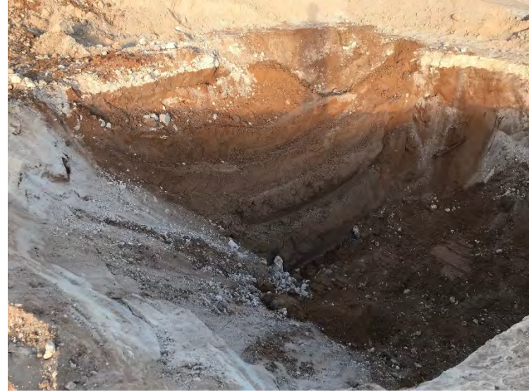
Photograph 2: View of open excavation near pothole PH04.
