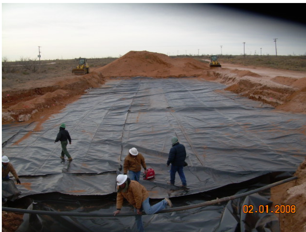
Photograph No. 11 – Installation of 20-mil liner over entire excavation.
