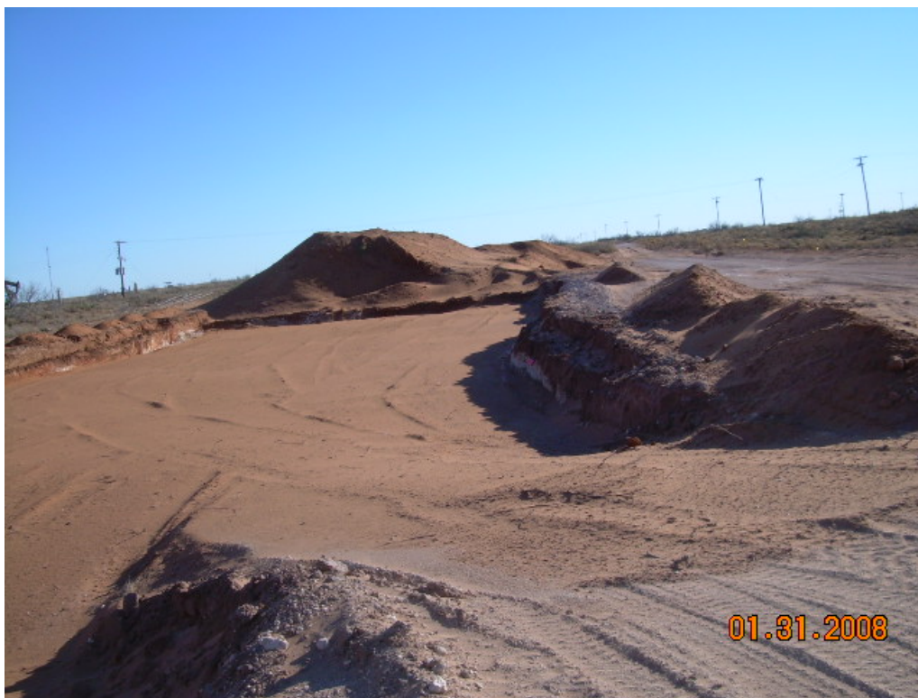
Photograph No. 8 – Looking southerly across excavation prepped for liner.
