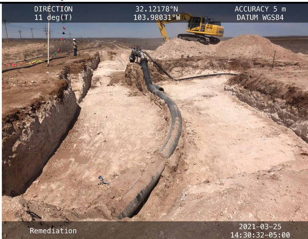
Photo 10: View of excavated release area, facing North. 3/25/2021
