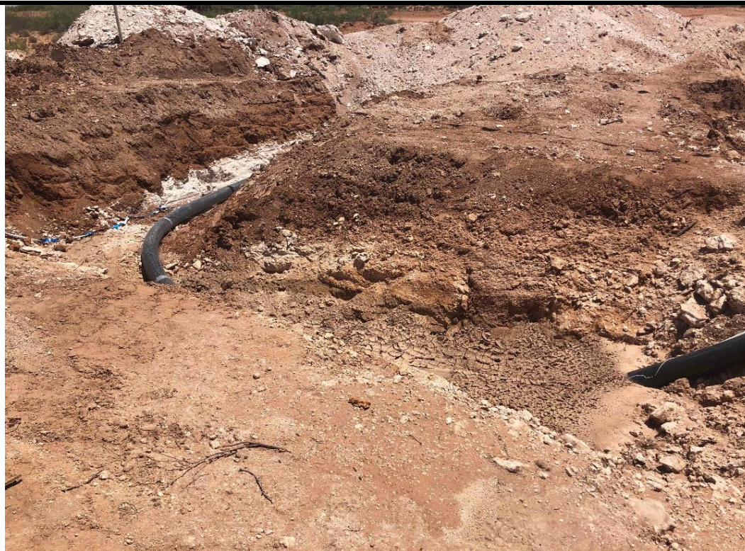
PHOTO 6: View of excavation east of release, facing Southeast. 7/6/2020
