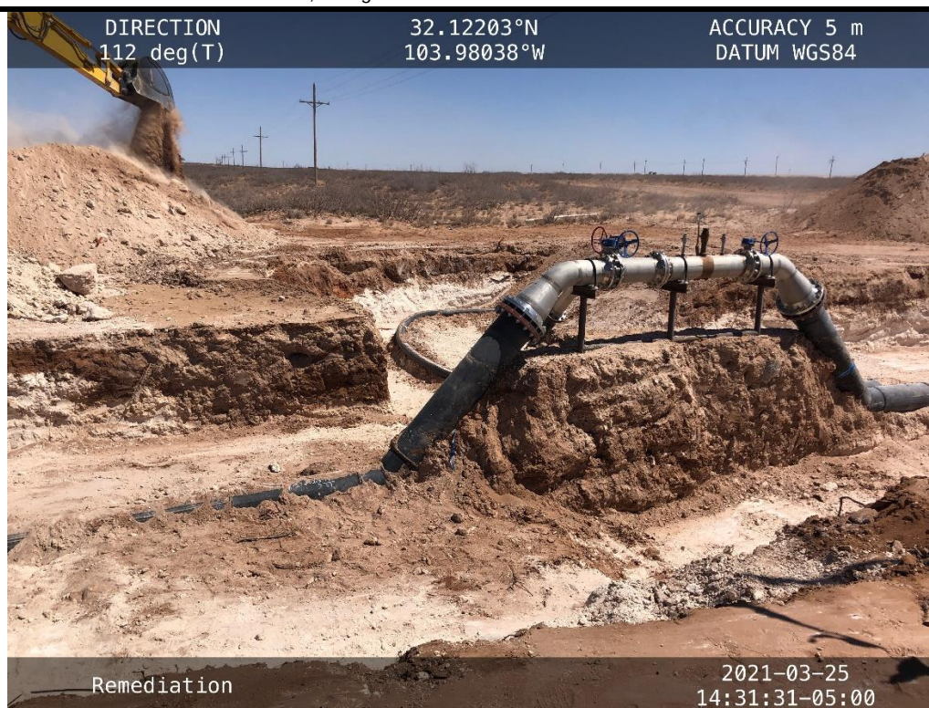
Photo 12: View of excavated release area, facing East. 3/25/2021
