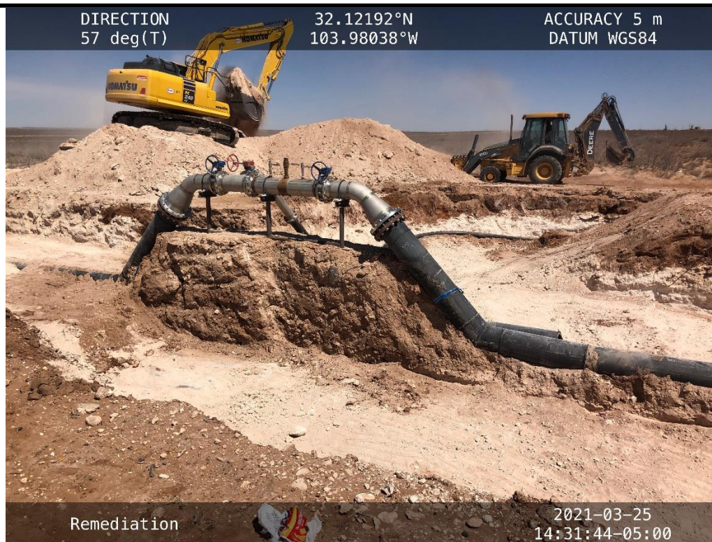
PHOTO 13: View of excavated release area, facing Northeast. 3/25/2021
