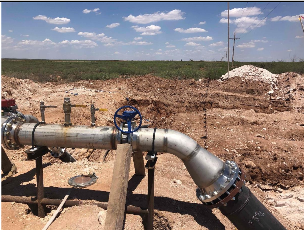
PHOTO 3: View of pipe junction installation, facing East. 7/6/2020
