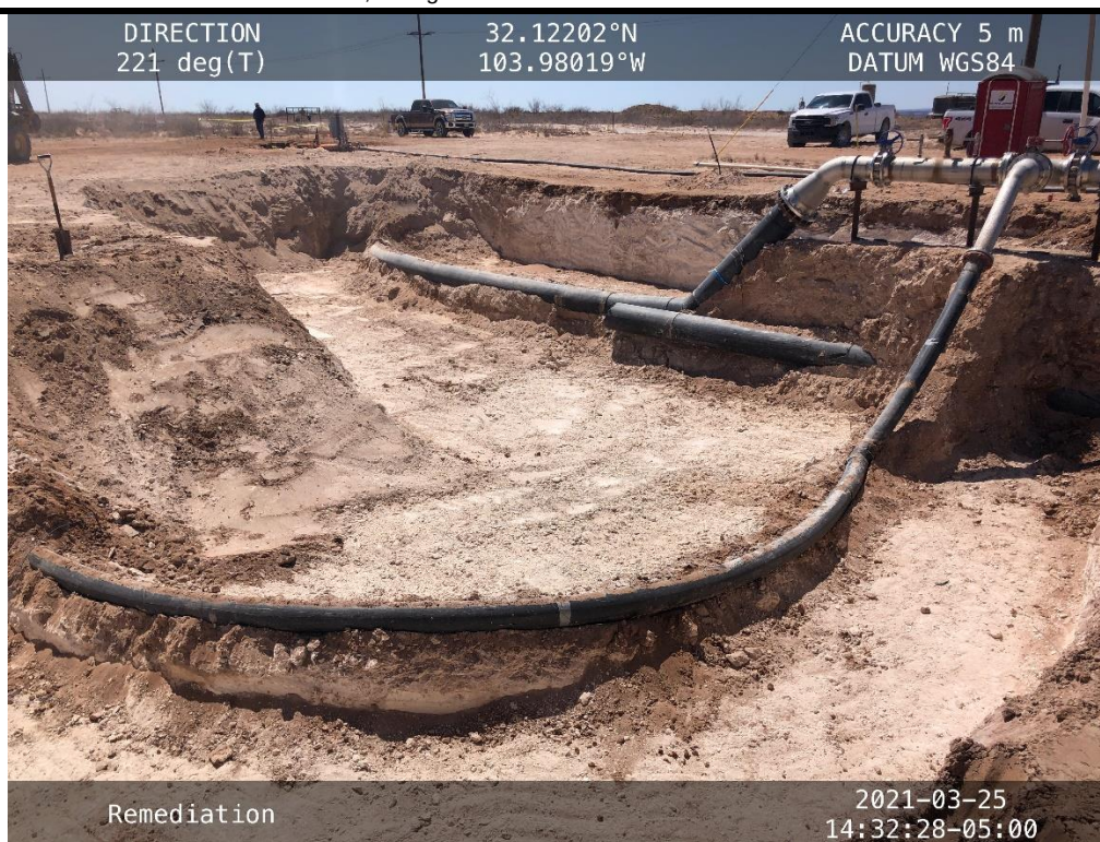
Photo 14: View of excavated release area, facing Southwest. 3/25/2021
