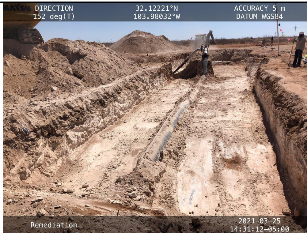
PHOTO 11: View of excavated release area, facing Southeast. 3/25/2021
