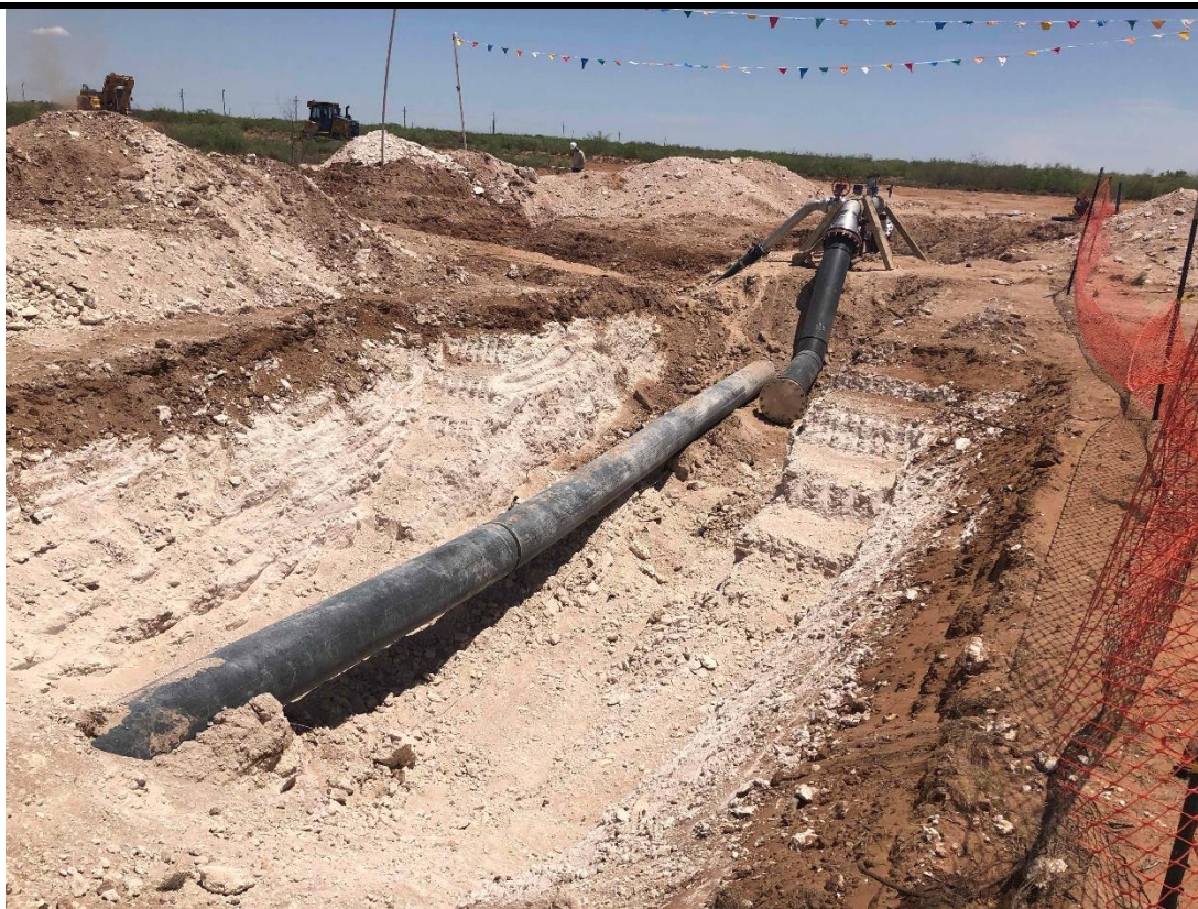
PHOTO 5: View of northern excavation, facing Southeast. 7/6/2020
