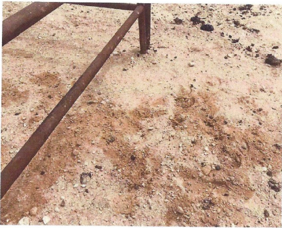
Staining outside of wellhead guard rail.
