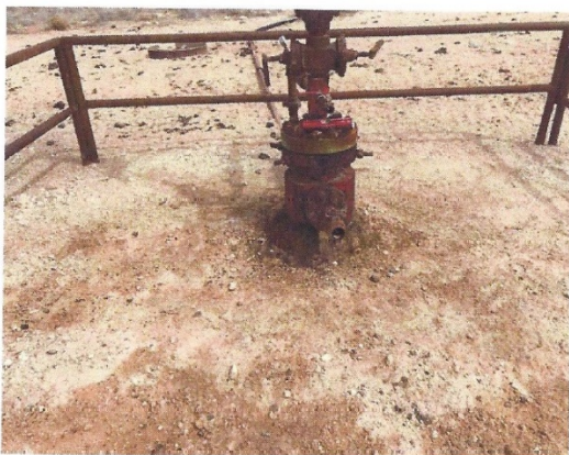
Picture of wellhead. Signs of release seeping through top layer of soil.
