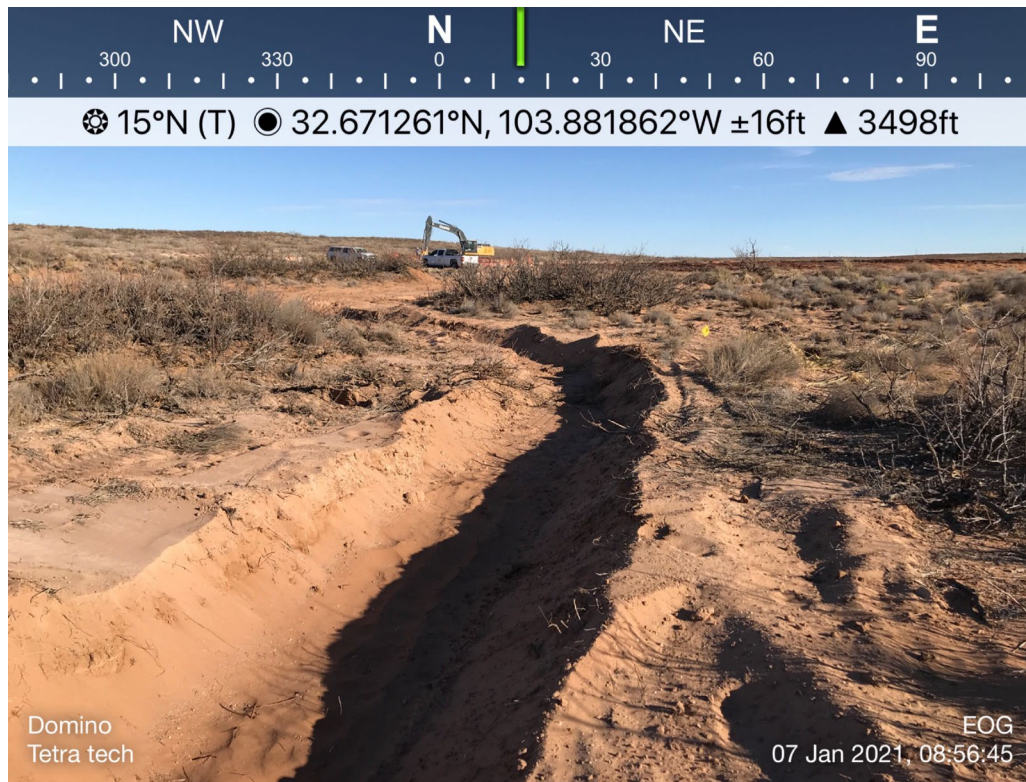
View North, area of Bottomholes 10 through 12
