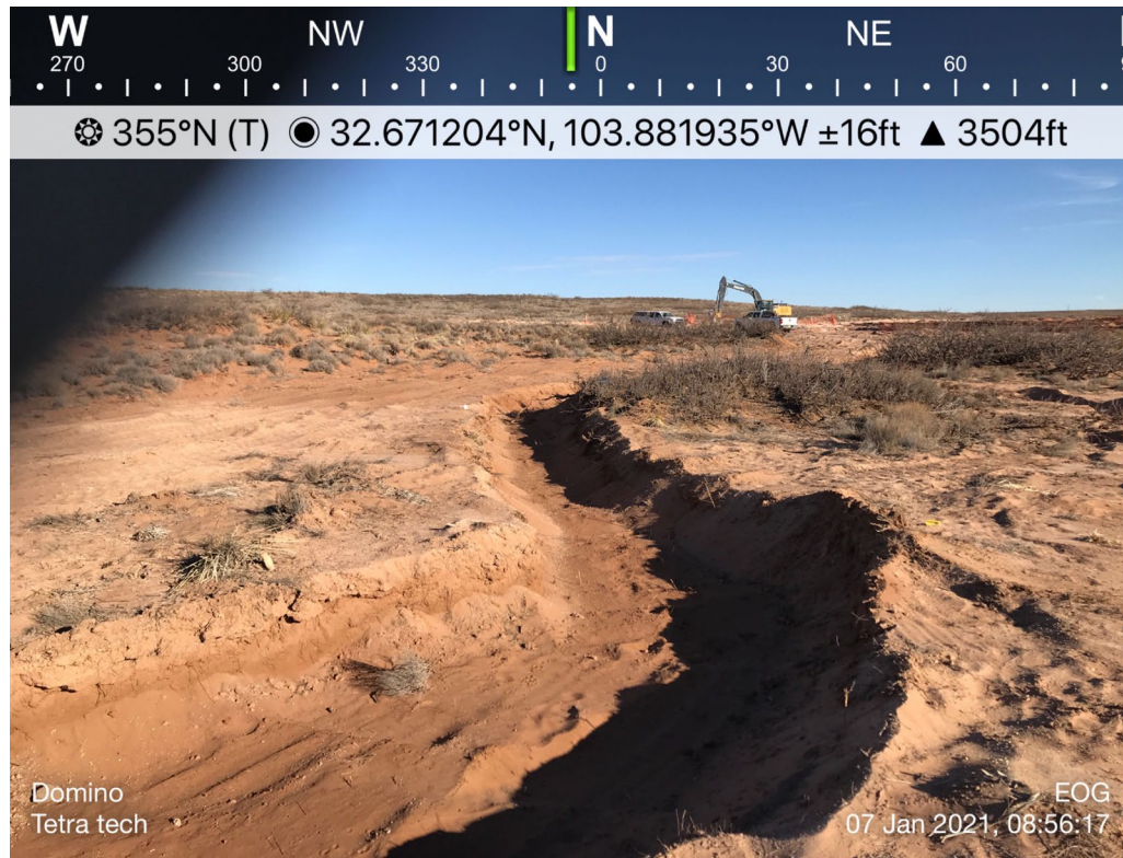
View North, area of Bottomholes 1 through 6
