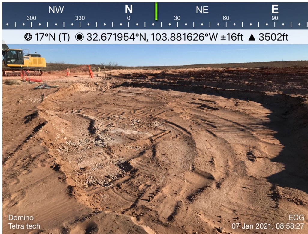
View North, area of Bottomholes 21 through 33
