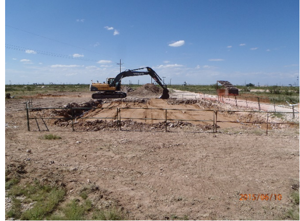
Padding the top of liner, facing north 6/10/2015
