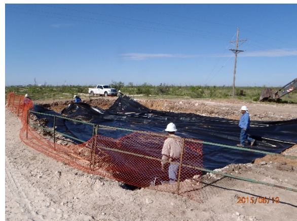
Installing 20-mil, reinforced liner, facing southwest 6/10/2015
