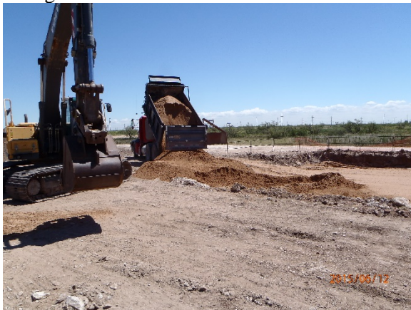
Backfilling with the excavation with imported blow sand, facing northeast 6/12/2015
