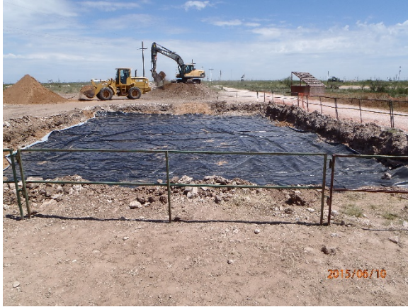
Liner is installed at 3.5 ft bgs, facing north 6/10/2015
