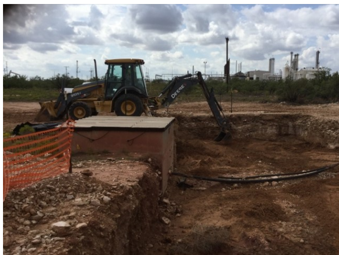
Padding excavation with imported blow sand, facing southeast
