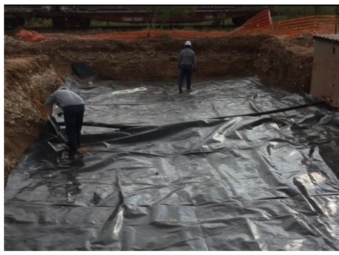
Installing and properly seating a 20-mil reinforced liner at 4.5 ft bgs, facing east
