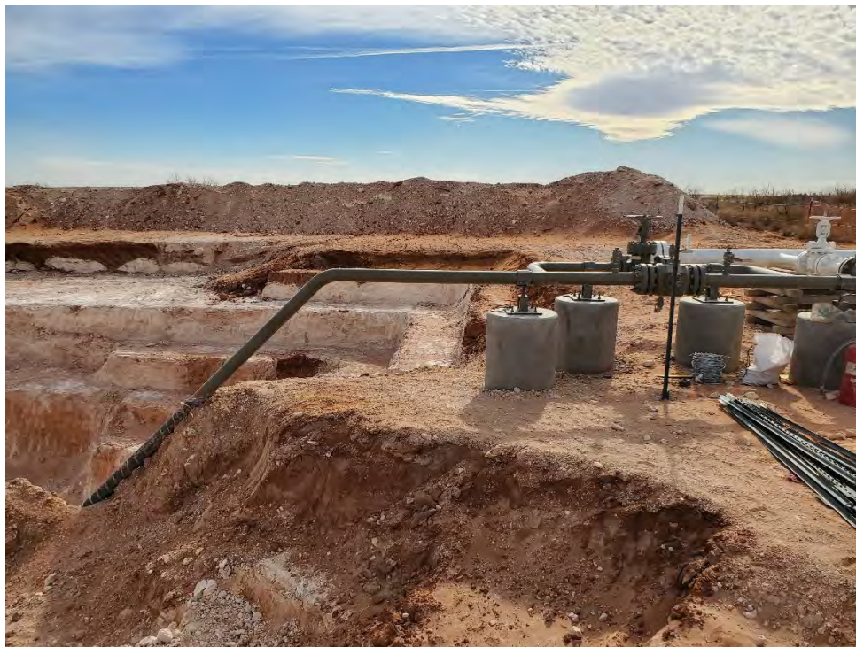
Photo 4 – Plains Riser and Pipeline on West Side of Excavation
