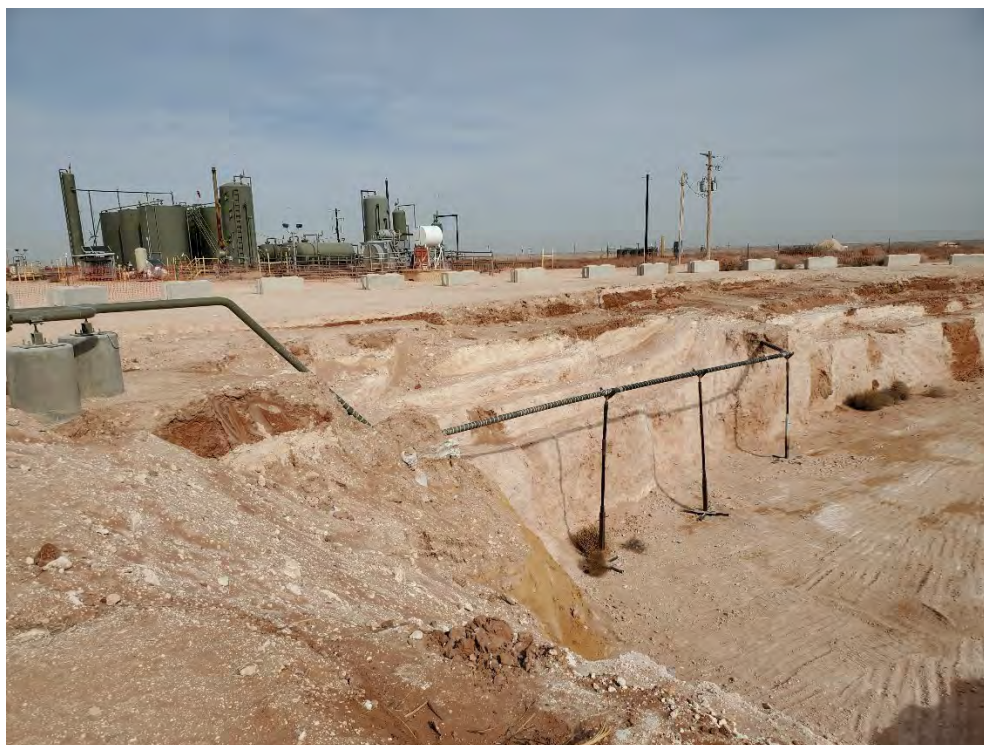
Photo 5 – Excavation Facing North with Conoco Phillips Pad in the Background
