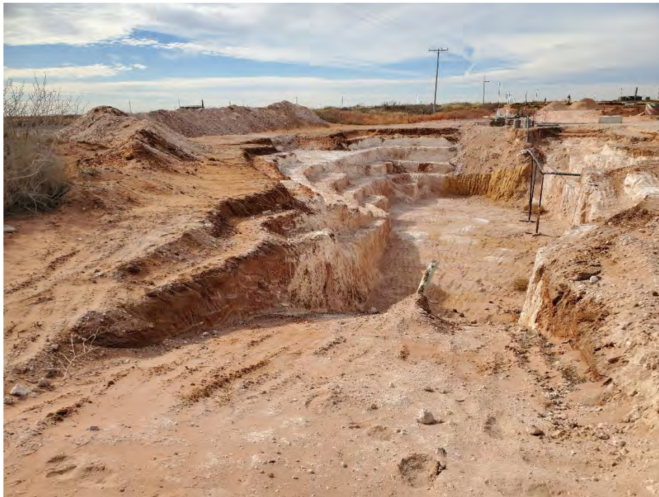
Photo 1 – Excavation Facing West
