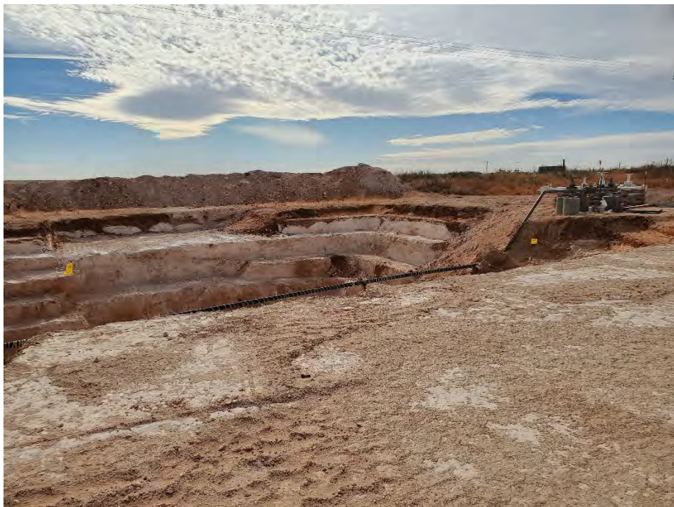
Photo 2 – Excavation Facing South
