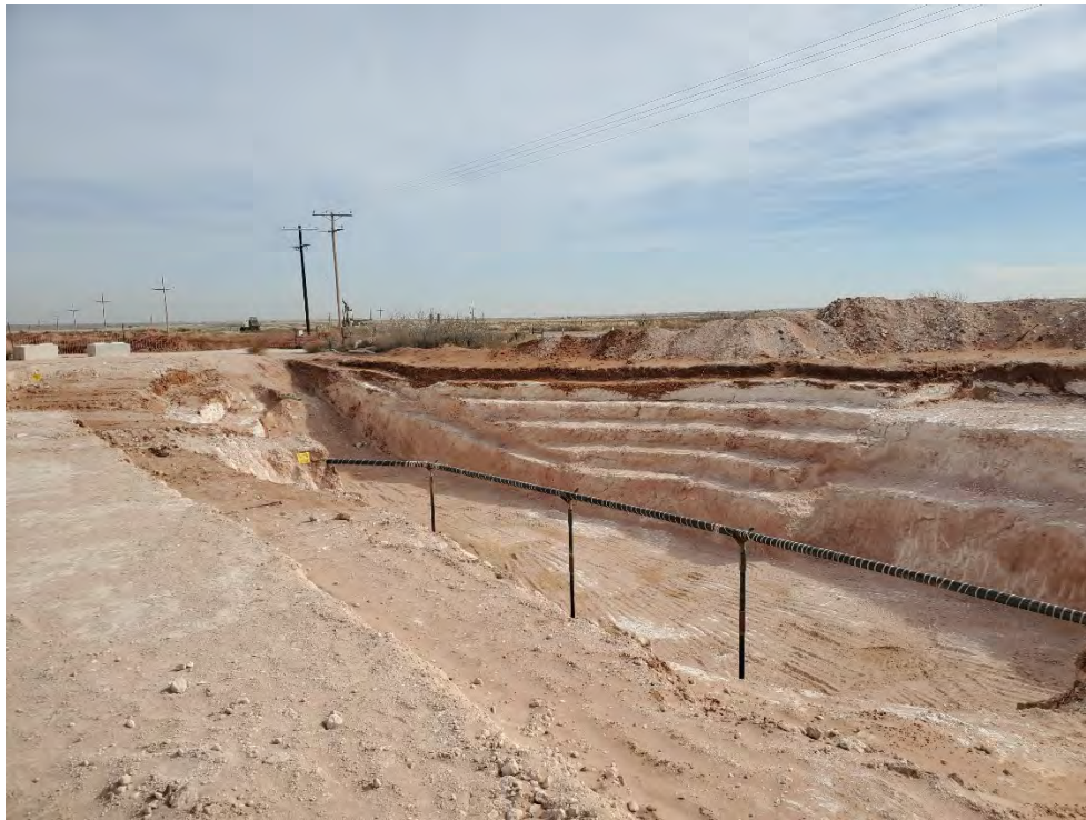
Photo 3 – Excavation Facing Southeast
