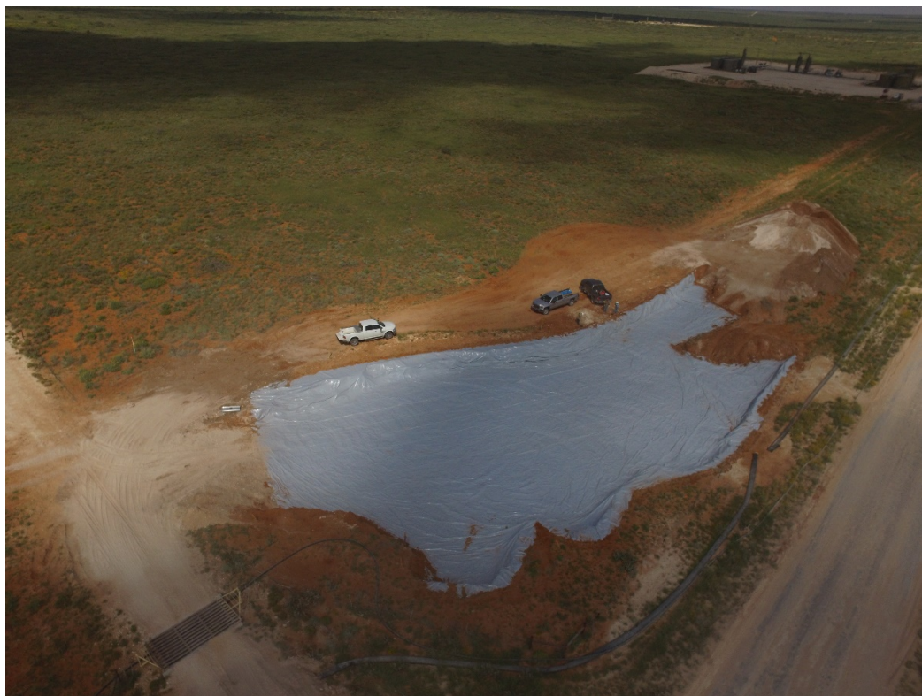
Figure 1: The liner was installed on the bottom and sides of the excavated area (photo taken from SE of spill).
