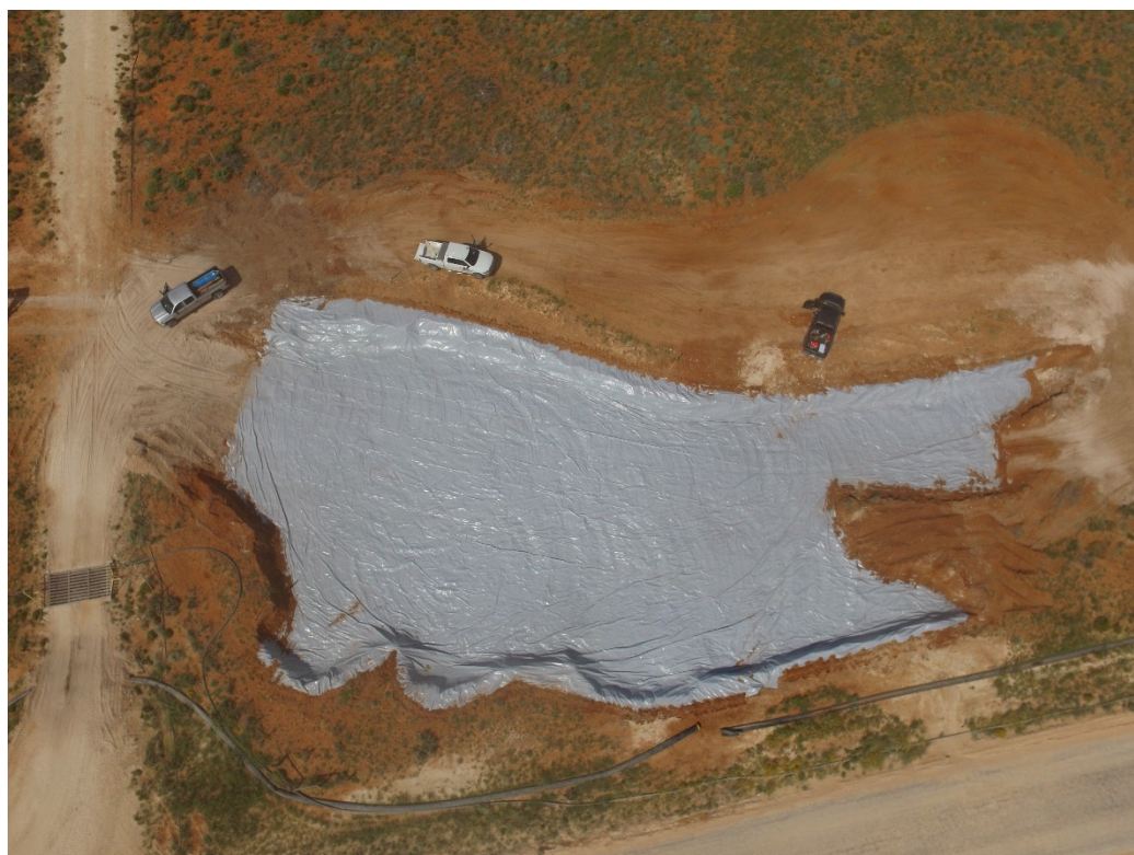
Figure 2: The liner was installed on the bottom and sides of the excavated area (photo taken from E of spill).
