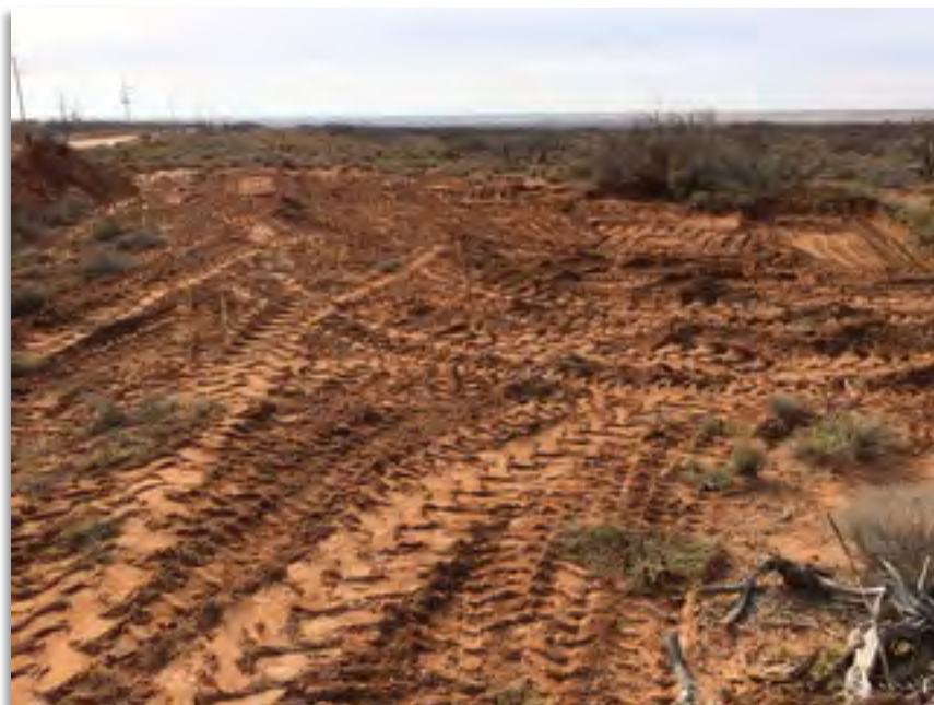
Figure 1: Initial release response excavation along the north-south pipeline. Stockpiled soil is visible photo left. GPS: 32.4284833 N, -103.6045694 W
