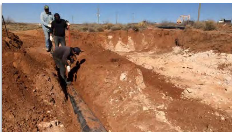
Figure 3: Excavation along the pipeline ROW. The pipeline is 4.5 feet below ground surface. Photograph is viewing north from the southern edge of Grid 4. Grid 5 is visible photo top right. GPS 32.428561 N, -103.6045389 W.
