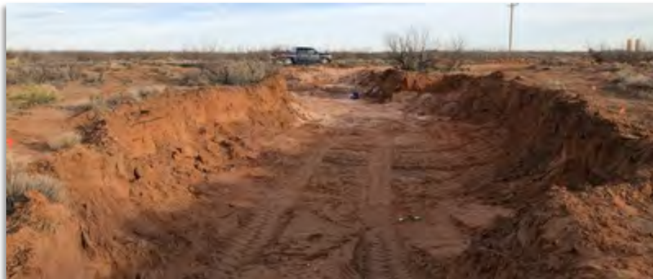
Figure 4: Photo of complete excavation prior to backfilling. Photo is viewing east from Grid 8 west wall. Excavation depth is 4.5-feet. GPS: 32.4286333 N, -103.6049278 W
