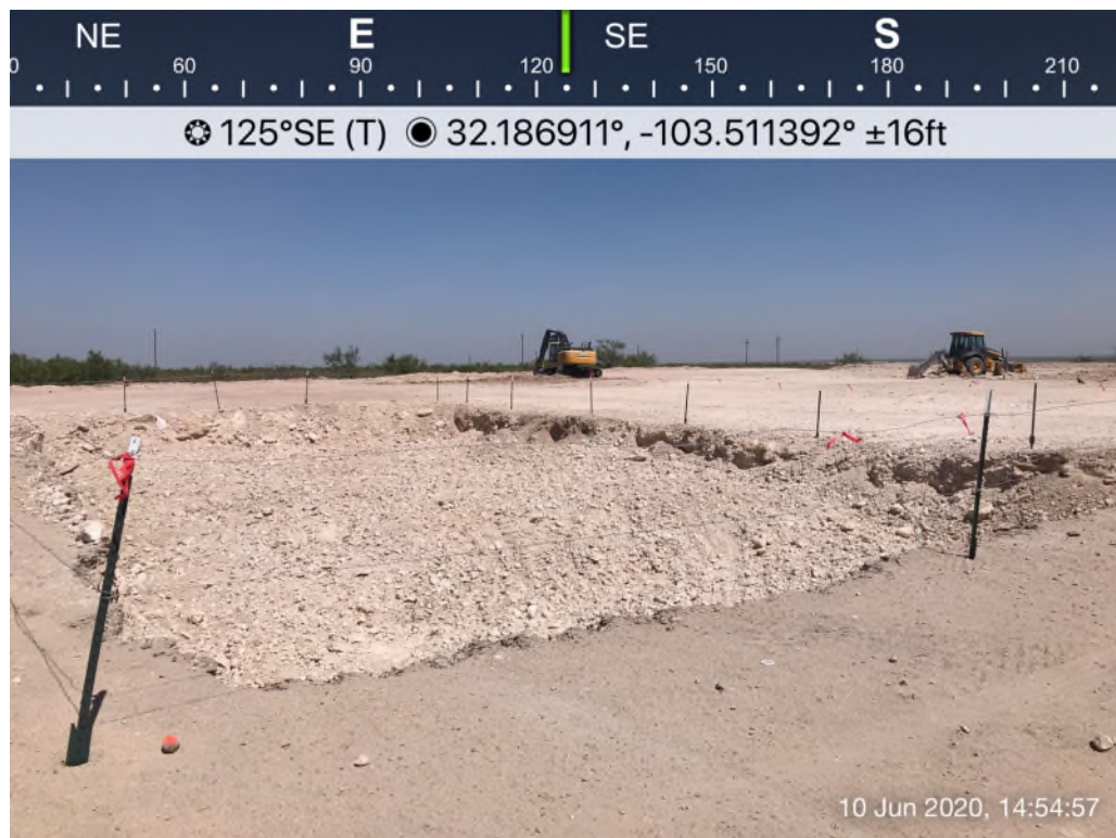
View of Remediation Activities – View Southeast
