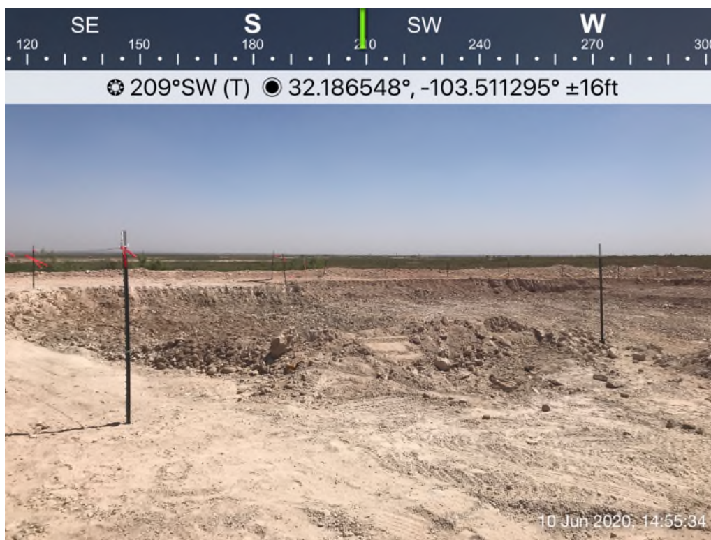
View of Remediation Activities – View Southwest
