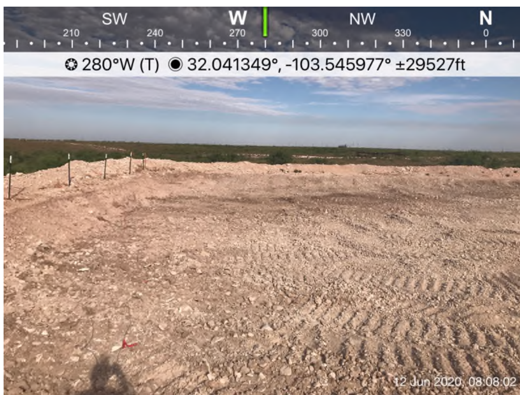
View of Remediation Activities – View West
