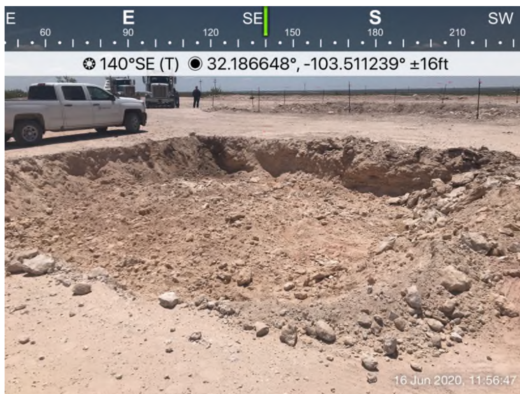
View of Remediation Activities – View Southeast
