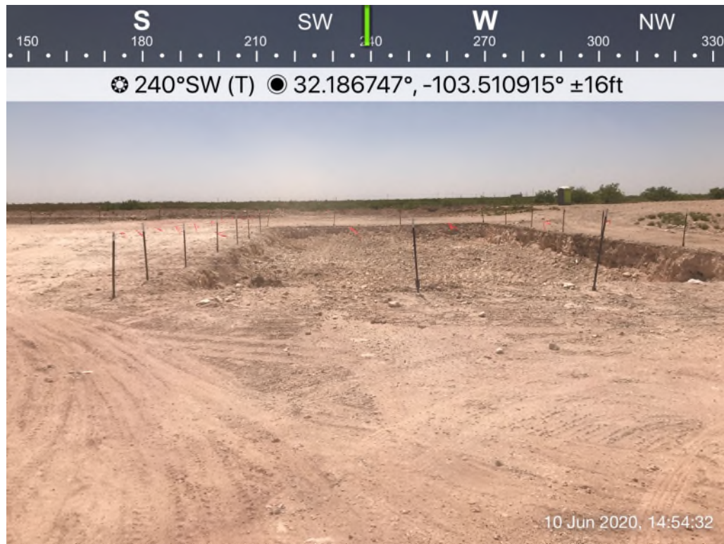
View of Remediation Activities – View Southwest
