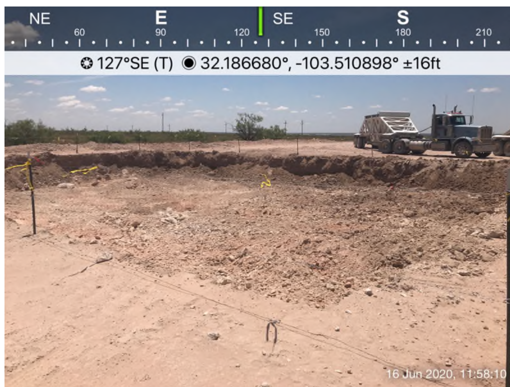
View of Remediation Activities – View Southeast
