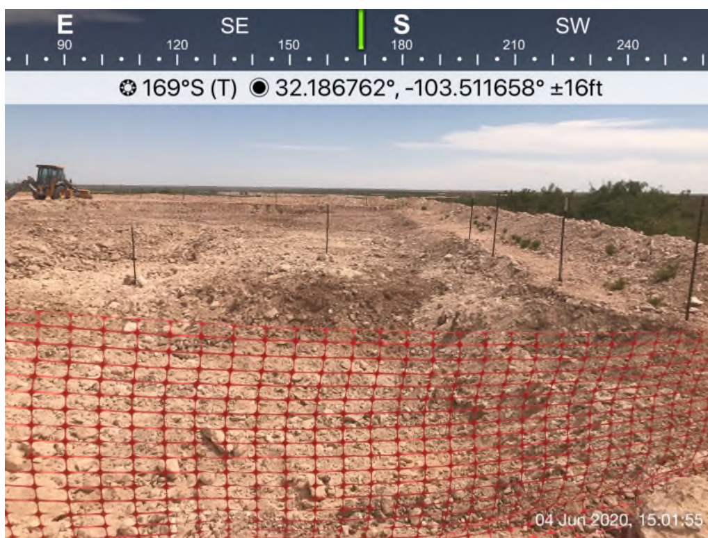
View of Remediation Activities – View South
