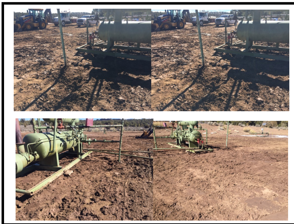
Site Area: Backfill February 11, 2021
