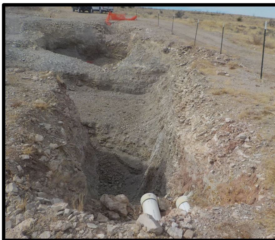
PHOTOGRAPH NO. 8 – A view of the pipeline area upon completion of the remedial process. The view is towards the northwest. (Approximate GPS Coordinates: 32.590634, -104.581826)
