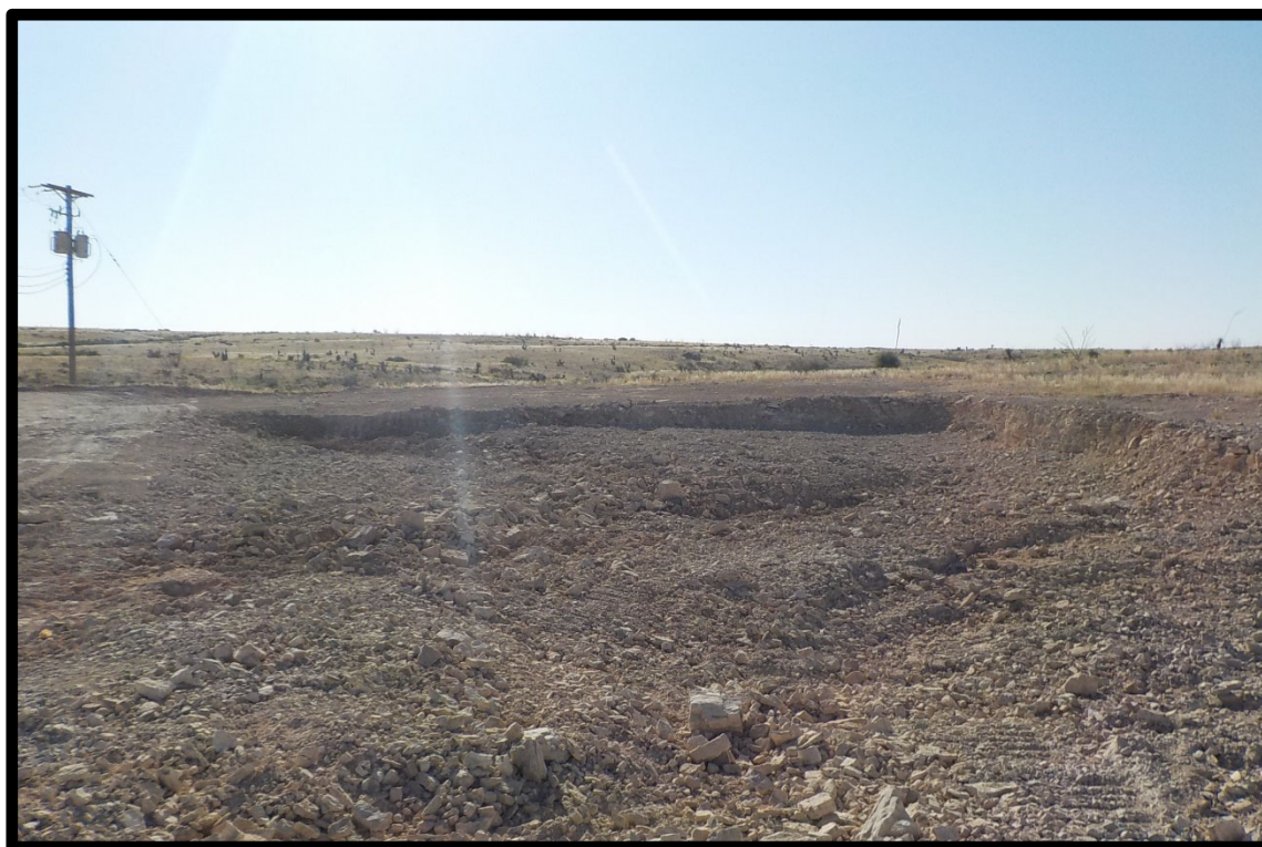
PHOTOGRAPH NO. 2 – A view of the tank battery area upon completion of the remedial process. The view is towards the west. (Approximate GPS Coordinates: 32.590593, -104.582195)
