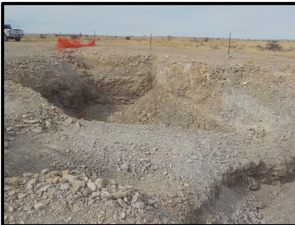
PHOTOGRAPH NO. 7 – A view of the western side of the pipeline area upon completion of the remediation process. The view is towards the northwest. (Approximate GPS Coordinates: 32.590598, -104.582062)
