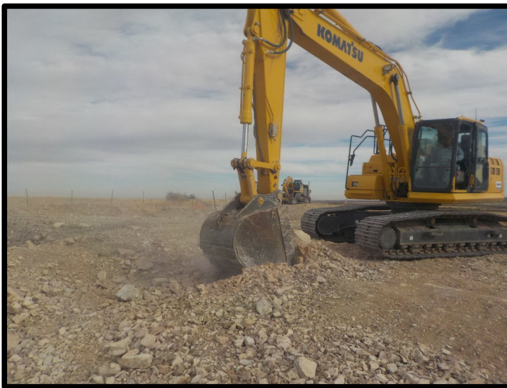
PHOTOGRAPH NO. 3 – A view of the remedial excavation activities on the facility pad area. The view is towards the east. (Approximate GPS Coordinates: 32.590491, -104.582411)
