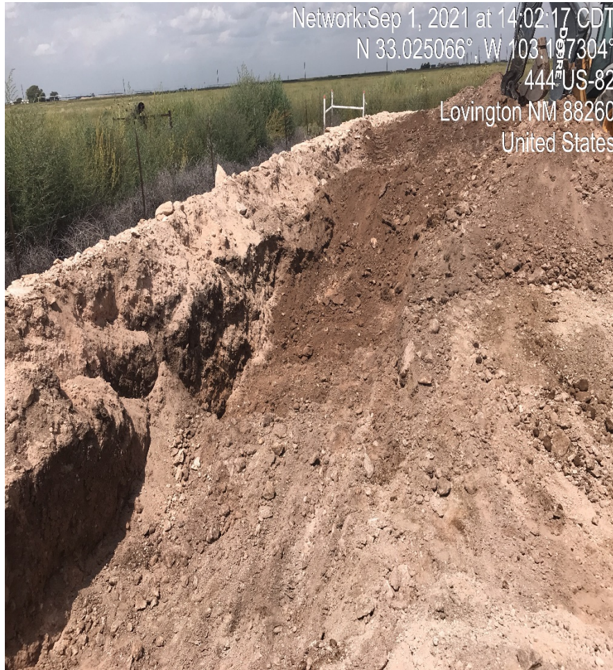
View North – Excavation activities conducted by the third-party contractor.
