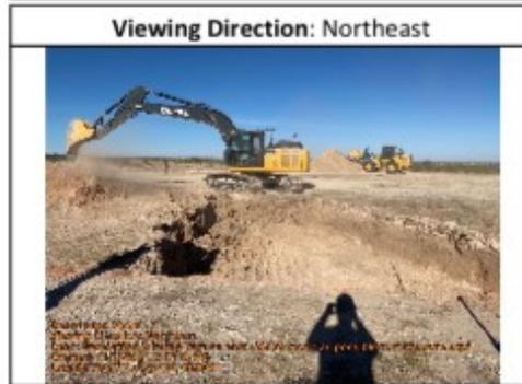
Excavation is being kept on east side as much as possible to make sure equipment can get to the pipeline when it is removed
