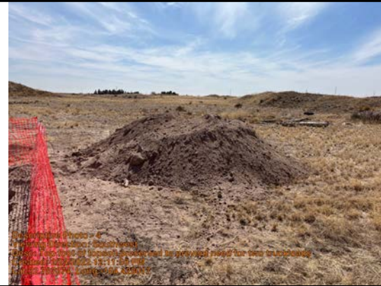
Top foot of clean topsoil preserved to prevent need for additional truckloads
