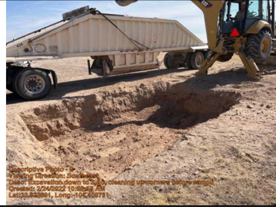
Excavation down to 3', cleaning up corners before sampling
