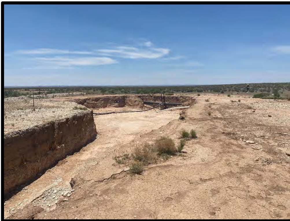
PHOTOGRAPH NO. 5 – A view of the Western Impact/Excavation Area collected during the EM Survey completed by Ranger on June 9, 2021. The view is towards the west-southwest. (Approximate GPS coordinates 32.682732, -104.499857)
