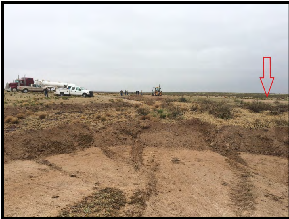
PHOTOGRAPH NO. 4 – An additional view of the April 12, 2016 release during the initial response activities. The view is from the northeastern extent of the impacted area towards the southwest. The Field Reported Agave Release Location (identified by the red arrow) can be seen in the photograph and is noted to be bare of vegetation. (Approximate GPS coordinates 32.682914, -104.499306)
