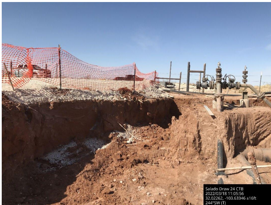
Excavated soil encompassing SW-6, March 18, 2022
