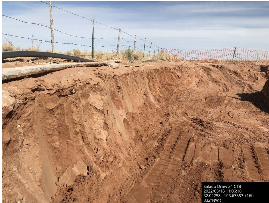
Excavated soil encompassing SW-1, March 18, 2022
