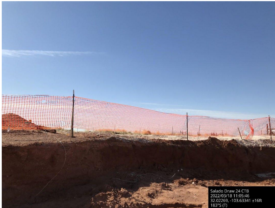
Excavated soil encompassing SW-5, March 18, 2022
