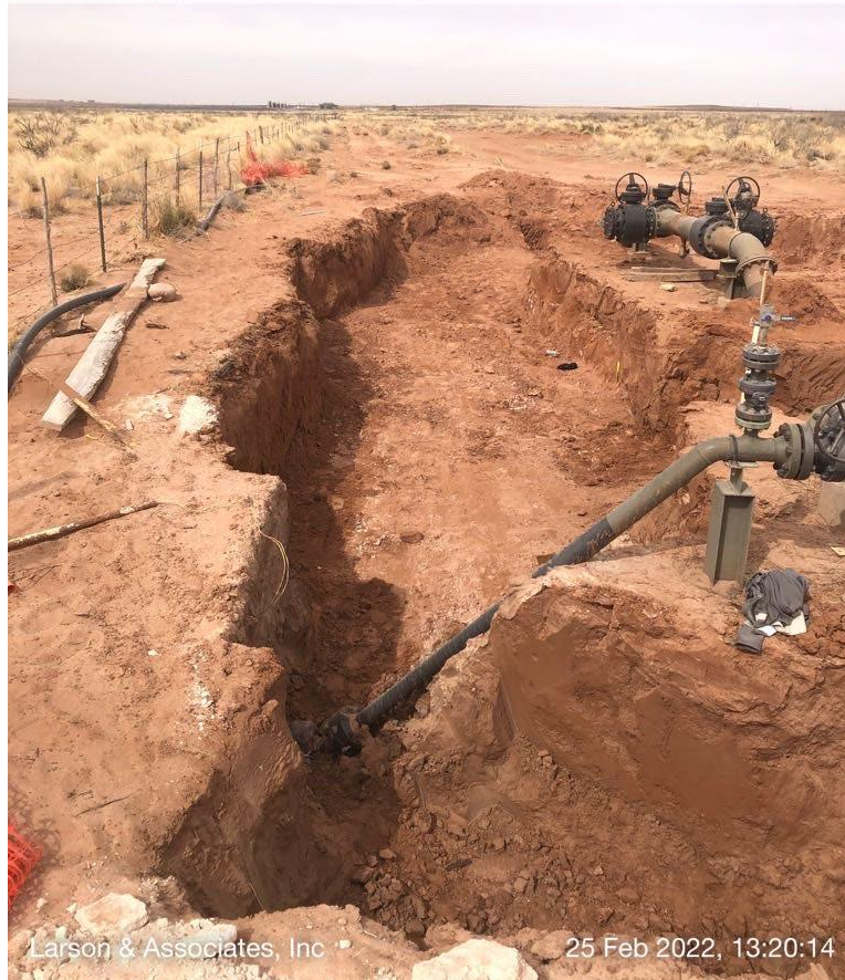
Excavated area viewing north, February 25, 2022
