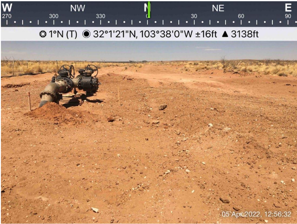
Seeded Excavation Area, April 5, 2022
