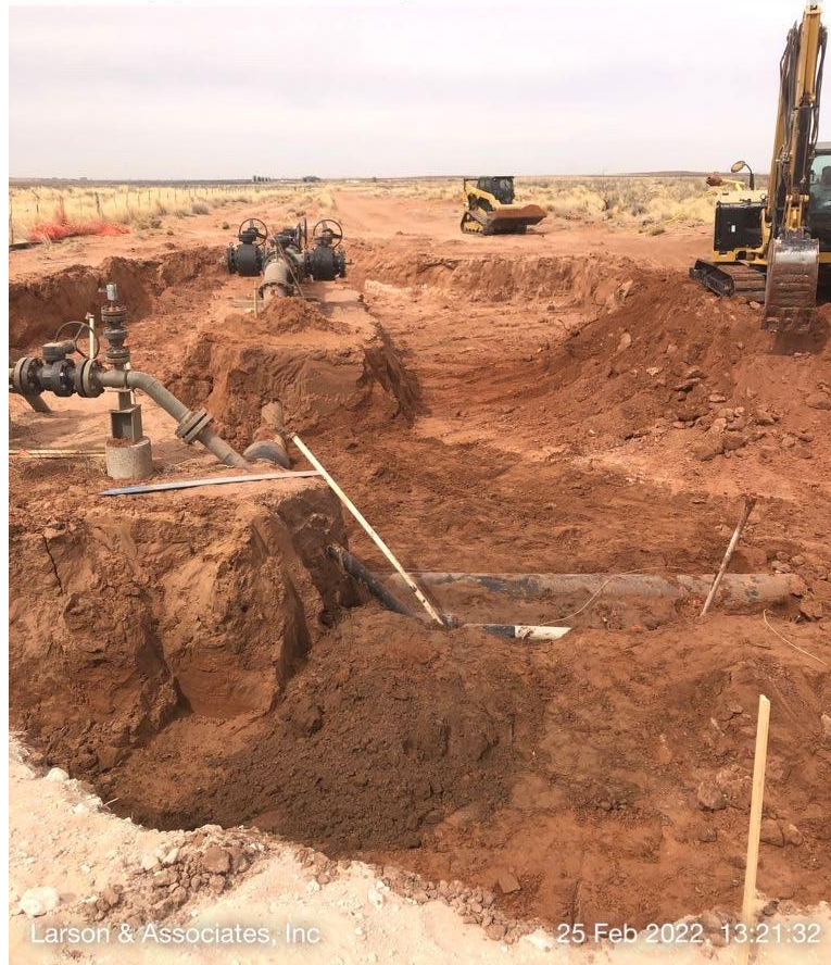
Excavated area viewing north, February 25, 2022
