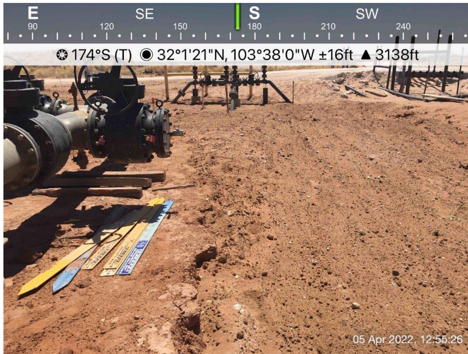
Seeded Excavation Area, April 5, 2022
