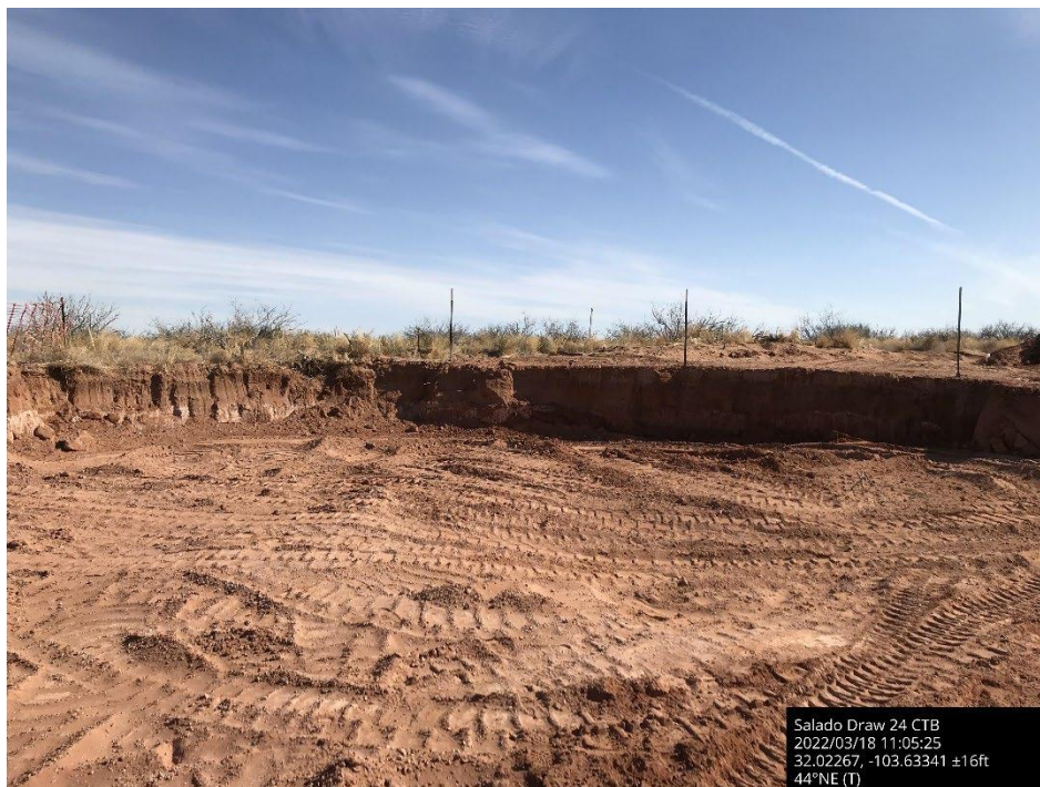
Excavated soil encompassing SW-3, March 18, 2022
