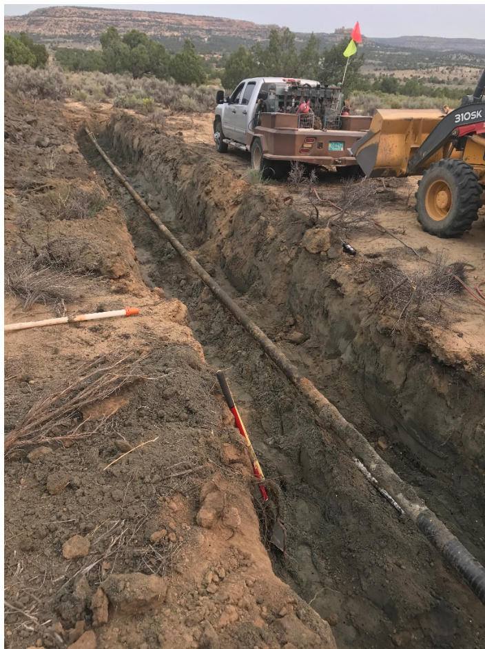
Photo 1: Excavation Around 4-Inch Pipe.
