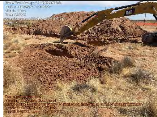
Bubbles out area where solidified oil material at surface at approximately 2' down
