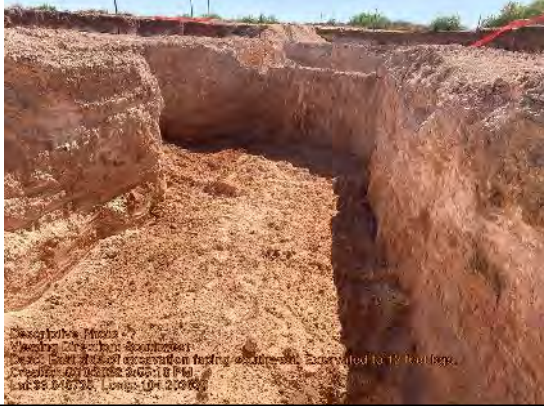
East side of excavation facing southwest. Excavated to 12 feet bgs.
