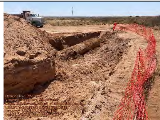
Southwest corner of excavation so far. Unearthed vertical heater treater in ground.
