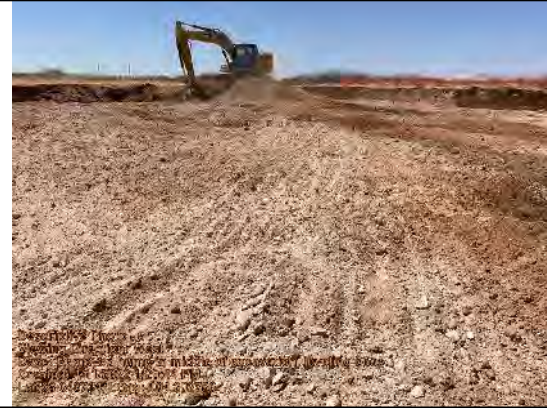
Removed hump in middle of excavation, leveling base to 4 feet bags.
