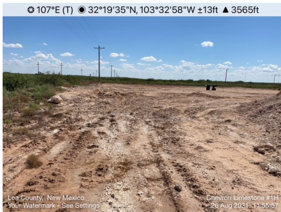
Impacted area viewing east, August 26, 2021
