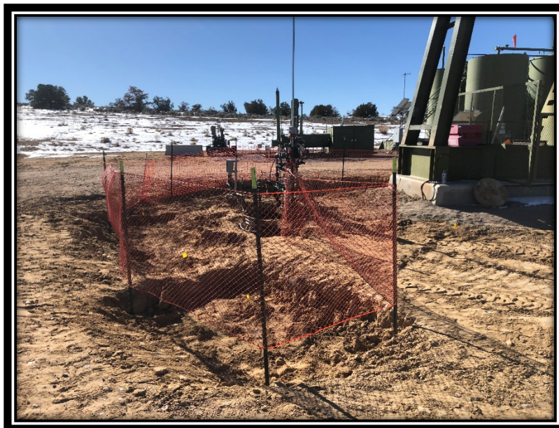
Picture 2: View of Excavations
