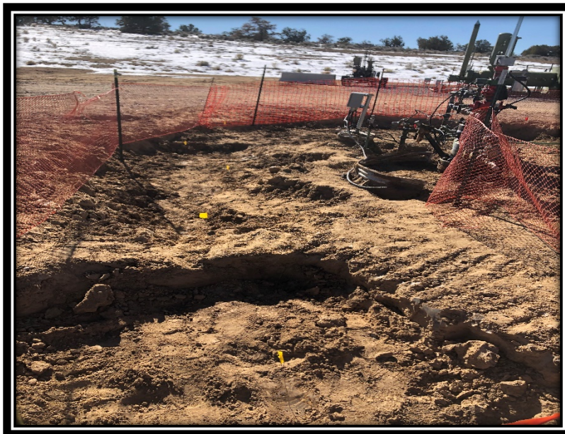
Picture 4: South Excavation with Sampling Points
