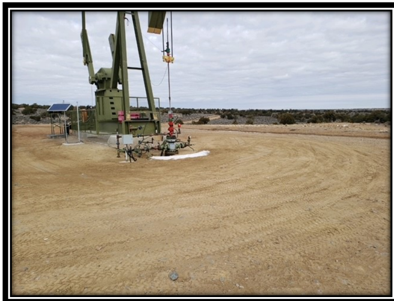
Picture 6: Backfilled and Recontoured Area
