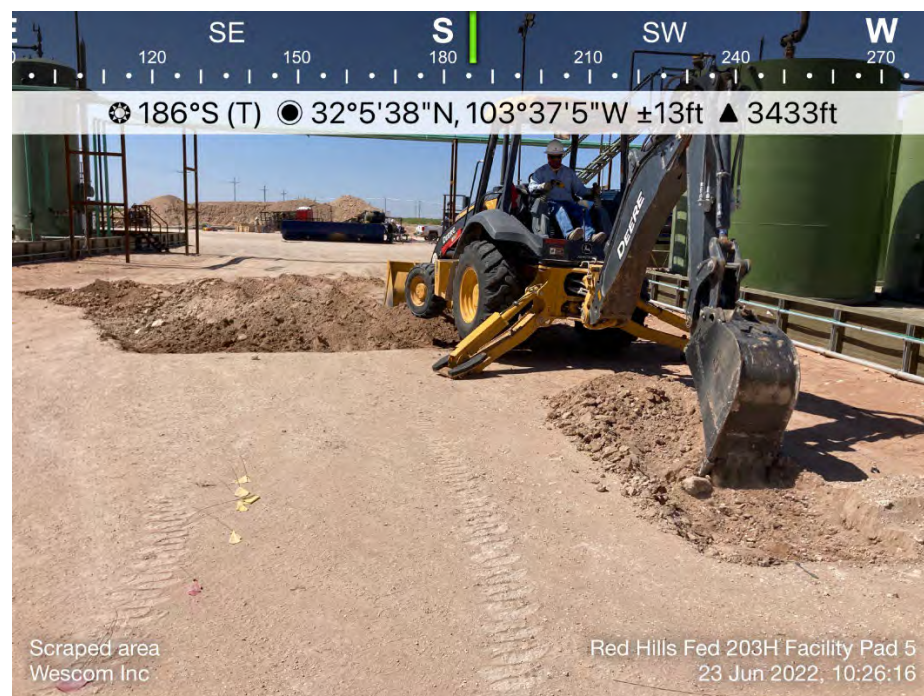
Excavation of Spill Area with Backhoe
