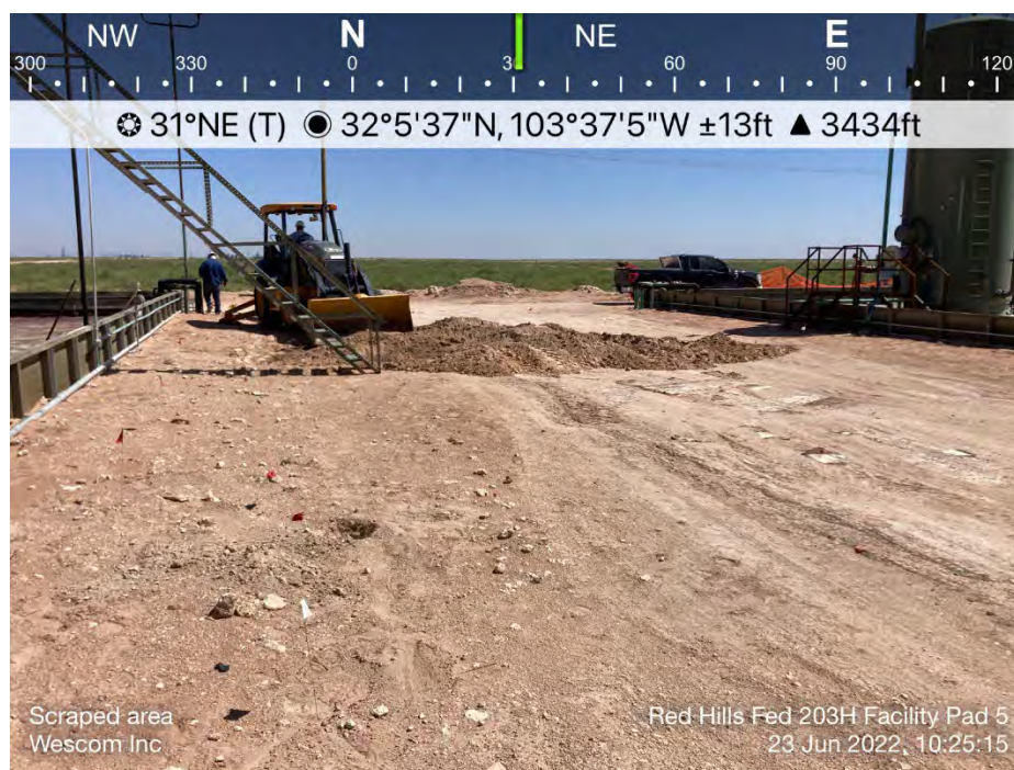
Excavation of Spill Area with Backhoe
