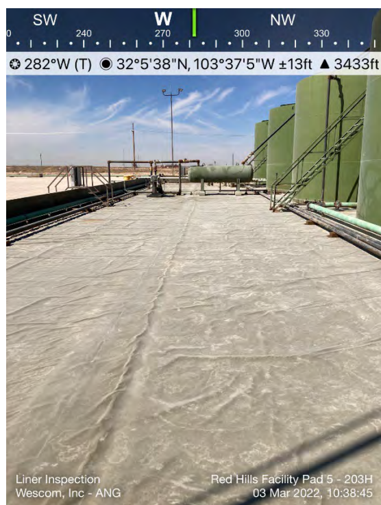
Tank Containment Liner Inspection South Side
