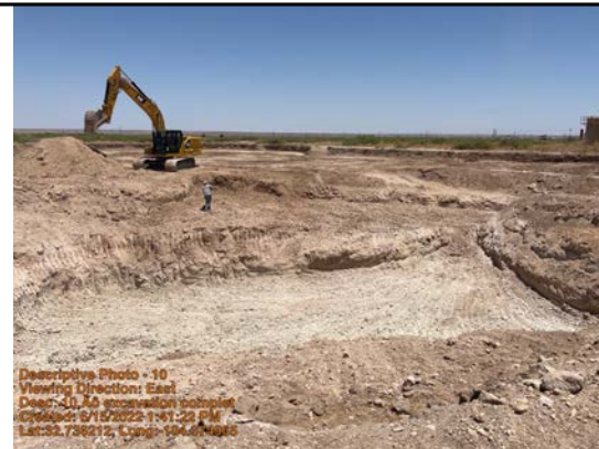
10' excavation completed
