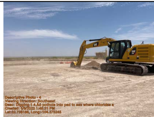
Digging 1.4' pothole into pad to see where chlorides are
