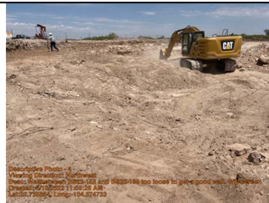
Wall between BS22-158 and BS22-168 too loose to get a good wall. Will screen this slope.
