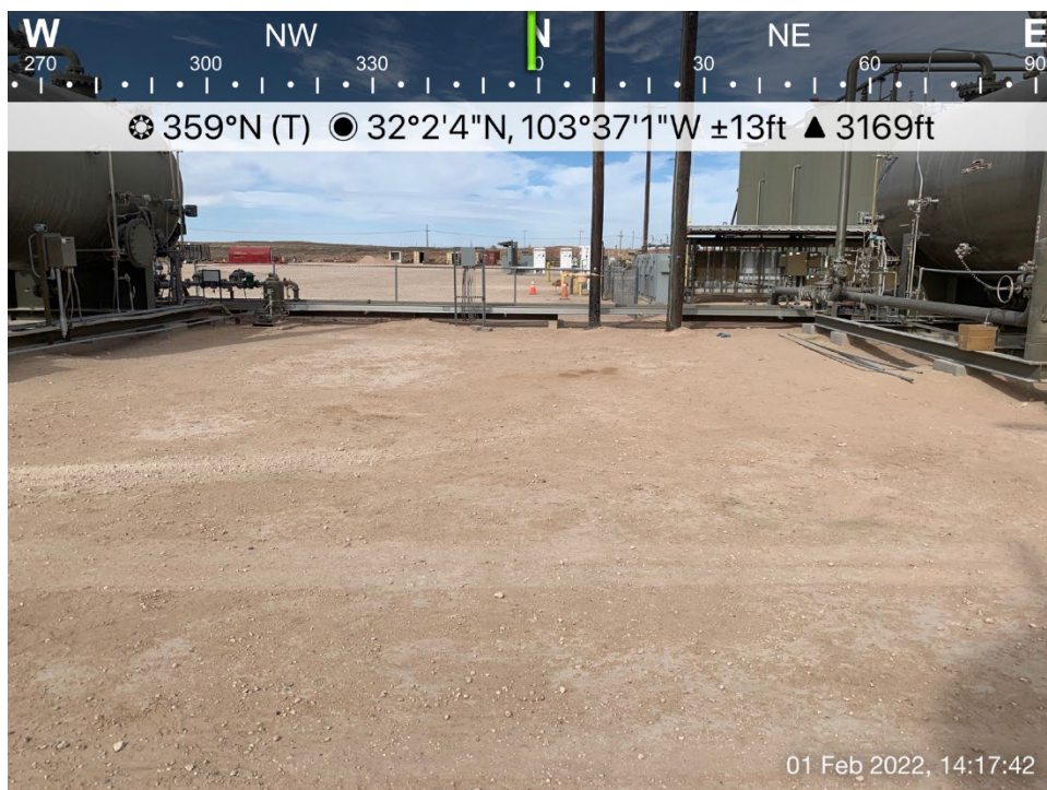
Waterline Release Impacted Area, Viewing North
