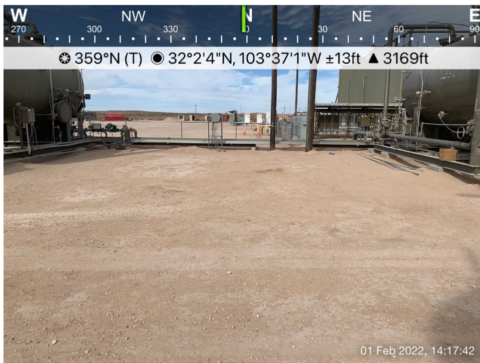
Waterline Release Impacted Area, Viewing North
