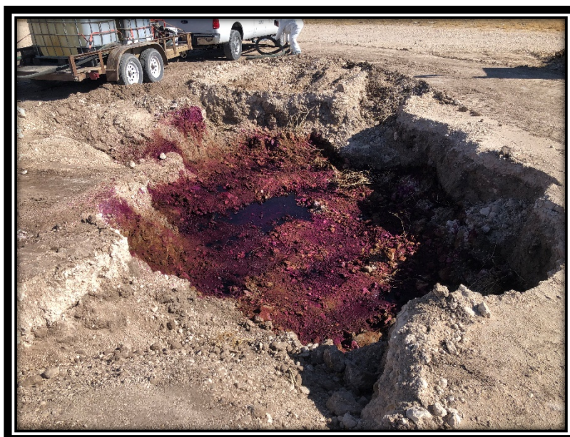
Picture 10: View of Potassium Permanganate Application
