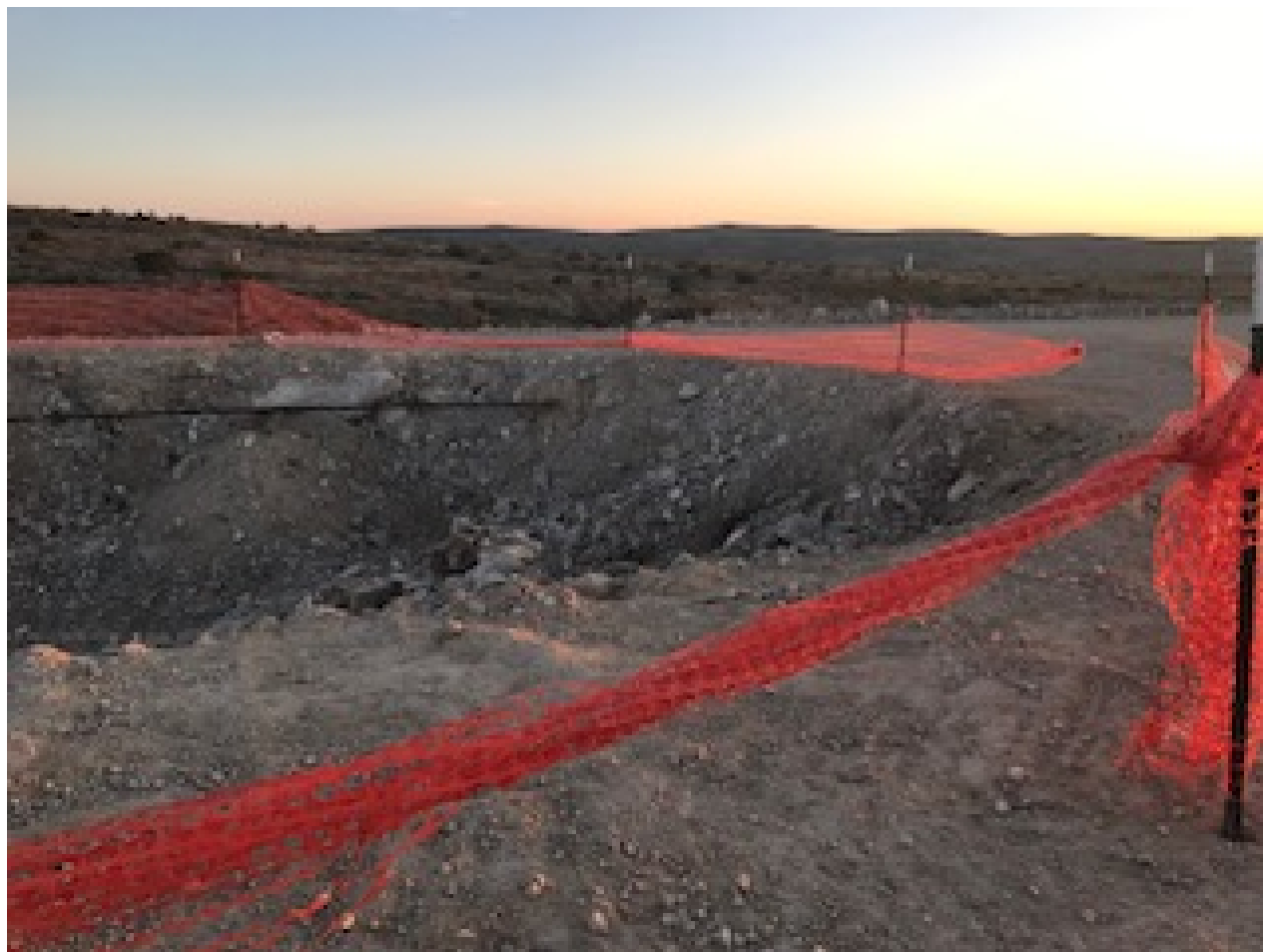
Excavation area – view north
