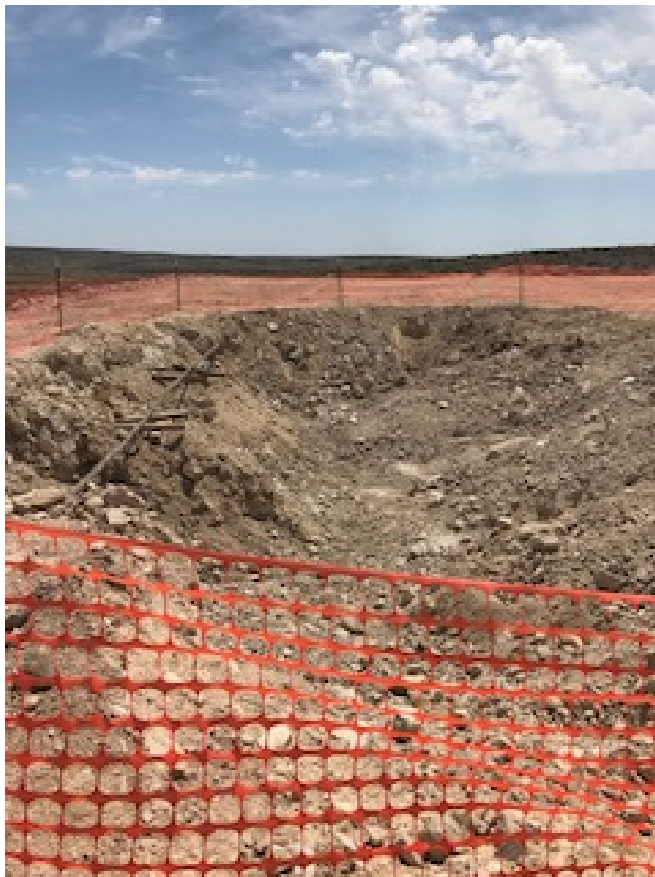
Excavation area – view northeast
