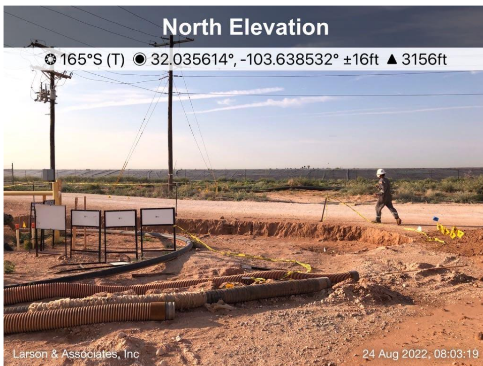
Excavated area viewing south, August 24, 2022
