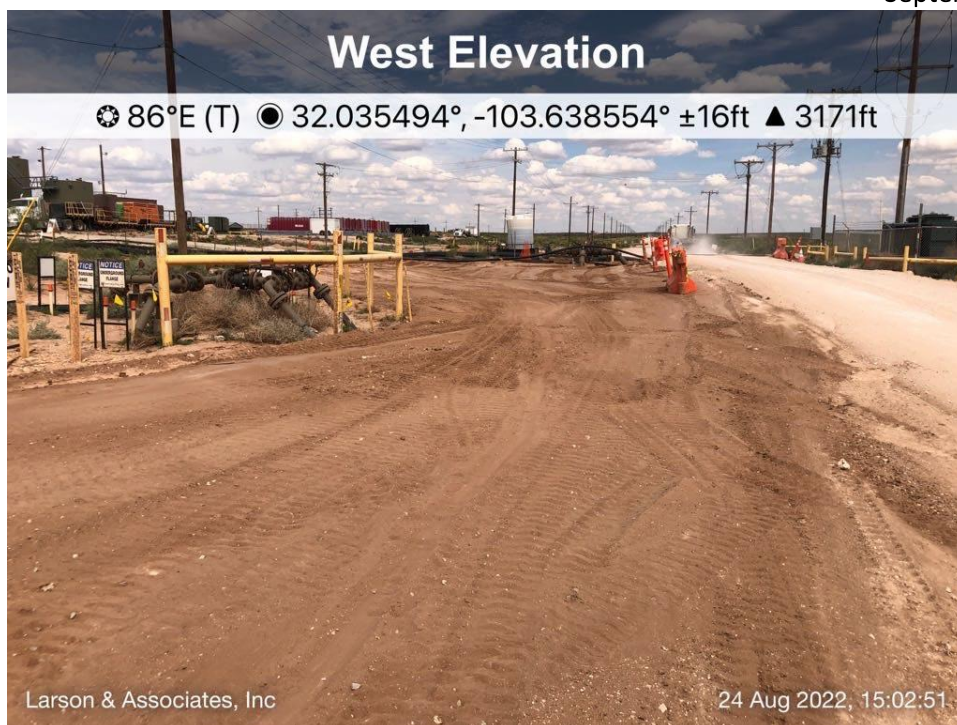
Excavation backfilled viewing east, August 24, 2022
