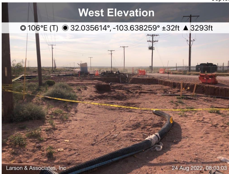
Excavated area viewing east, August 24, 2022
