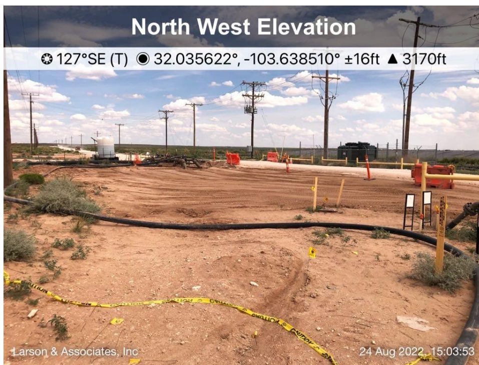
Excavation backfilled viewing southeast, August 24, 2022
