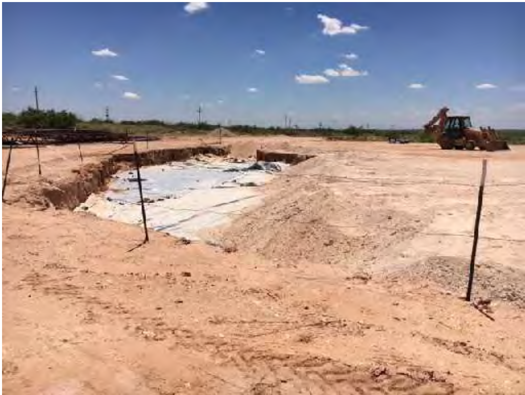
Photo 5: Liner installation and backfill of excavation facing southwest towards entrance
