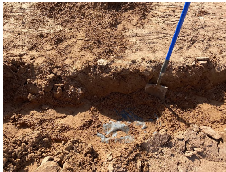
Photograph 4: Previously installed liner near SP-4 exposed.
