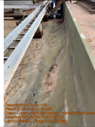
Liner within secondary containment (west wall)
