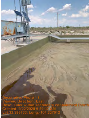
Liner within secondary containment (north wall)
