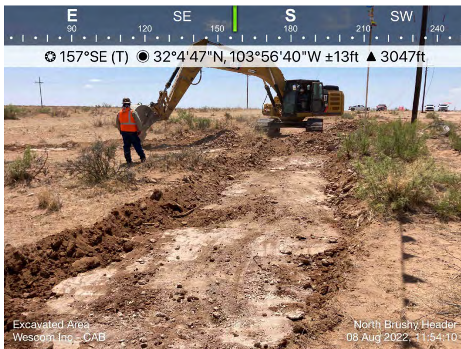
Excavation of Spill Area – North End
