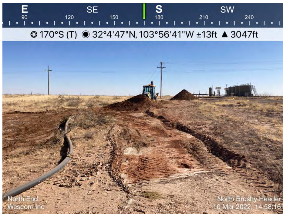
Initial Scrape and Contaminated Soil Pile
