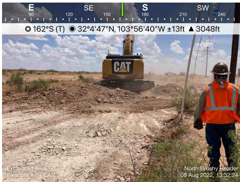
Excavation of Spill Area – Northeast Side
