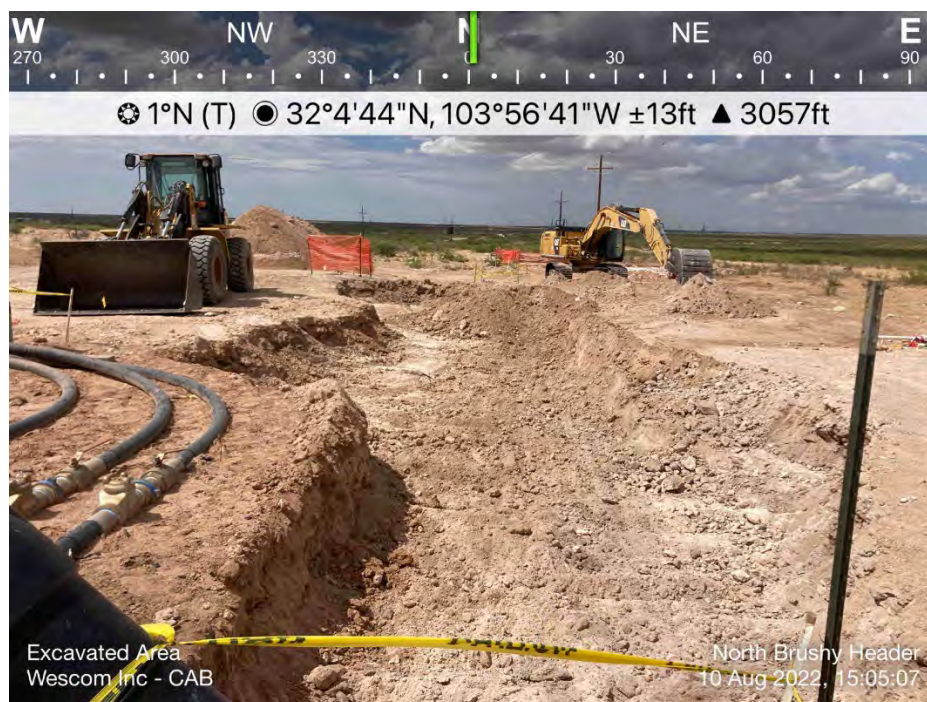
Excavation of Spill Area - South End
