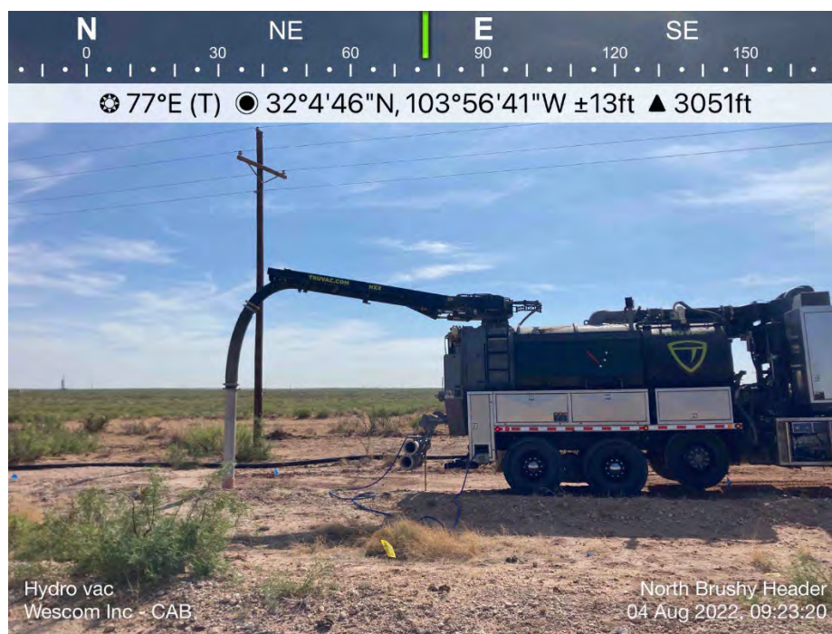
Hydrovac Water and Gas Lines
