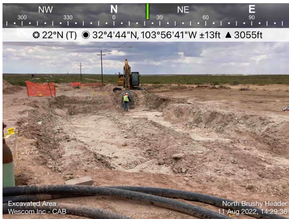
Excavation of Spill Area - South End
