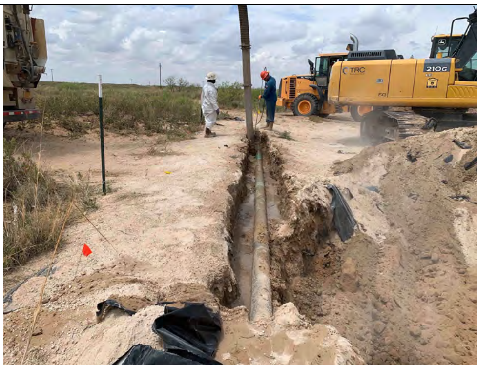
Photo 5: Hydro-excavating soil by pipeline.
