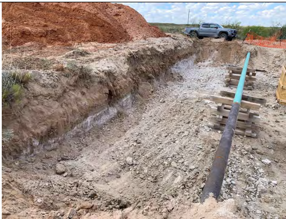
Photo 9: Finished excavating to 4.5 feet bgs.
