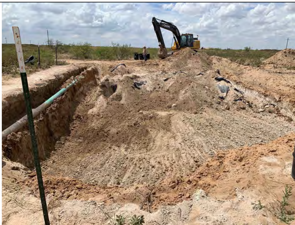
Photo 6: Excavating area to a depth of 4.5 feet below ground surface (bgs).
