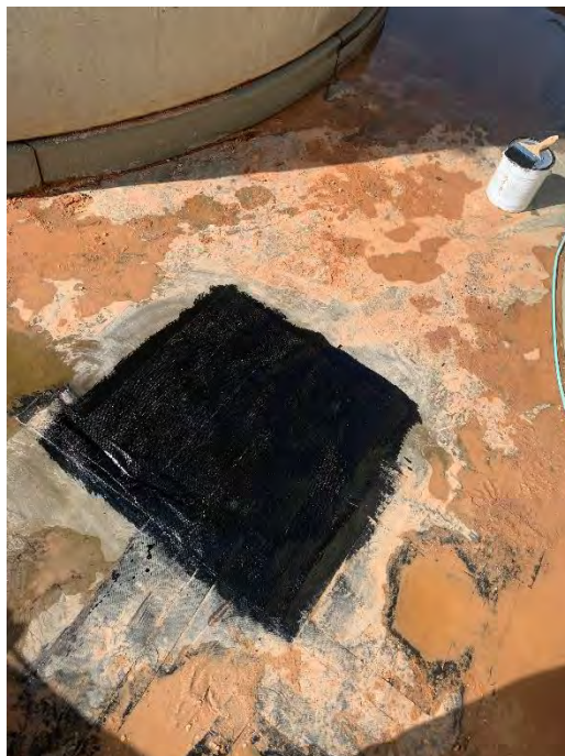
Liner Repaired (CONF06)
