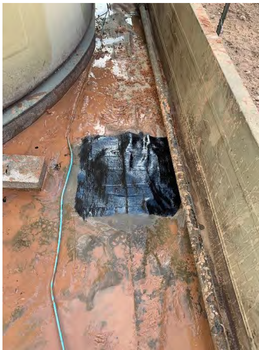
Liner Repaired (CONF07)
