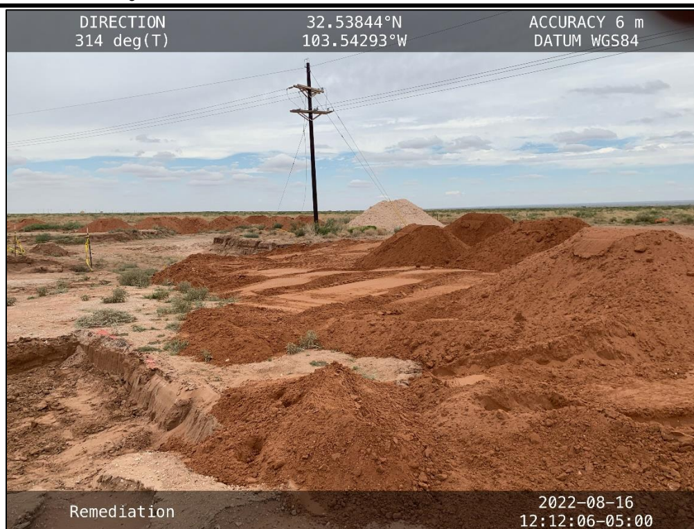
PHOTO 15: View of backfilling of excavation
