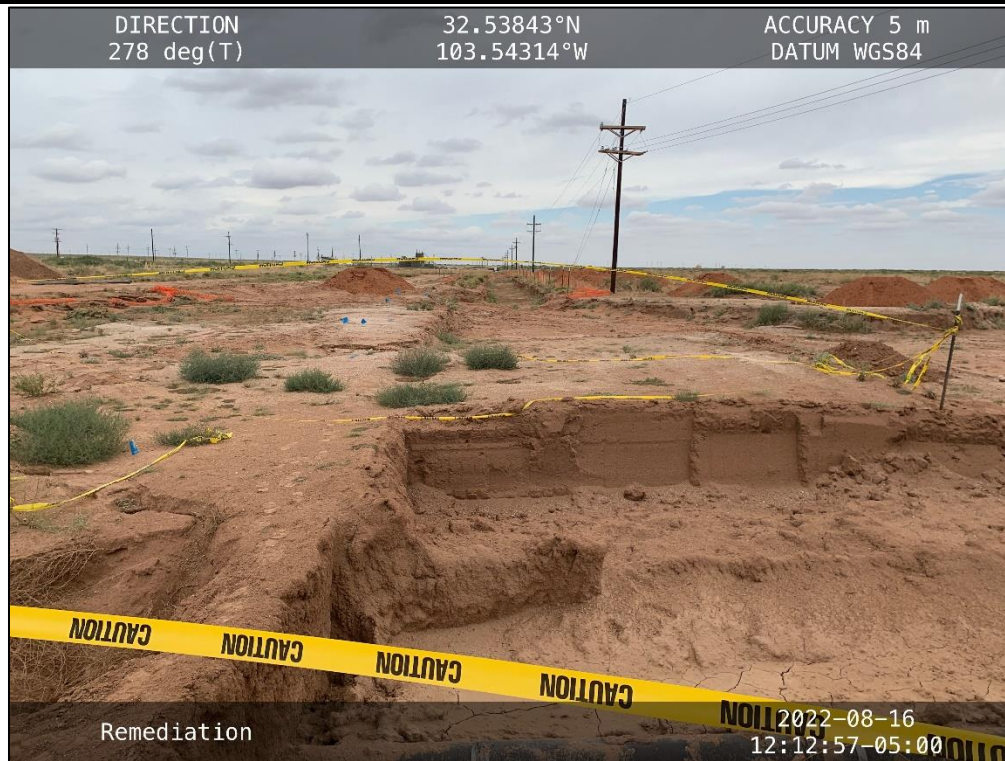
PHOTO 18: View of excavation
