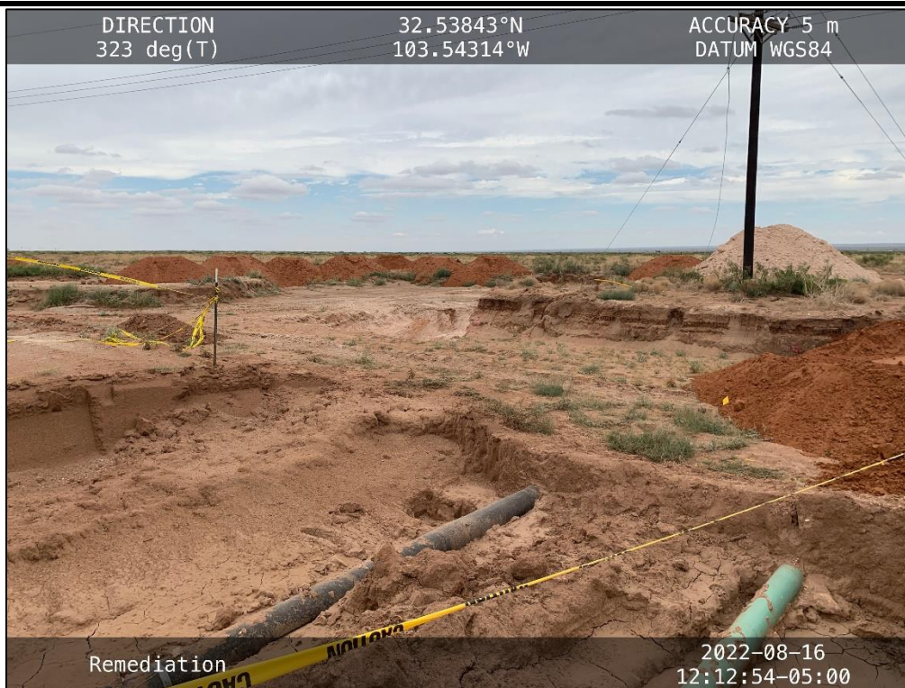
PHOTO 19: View of excavation
