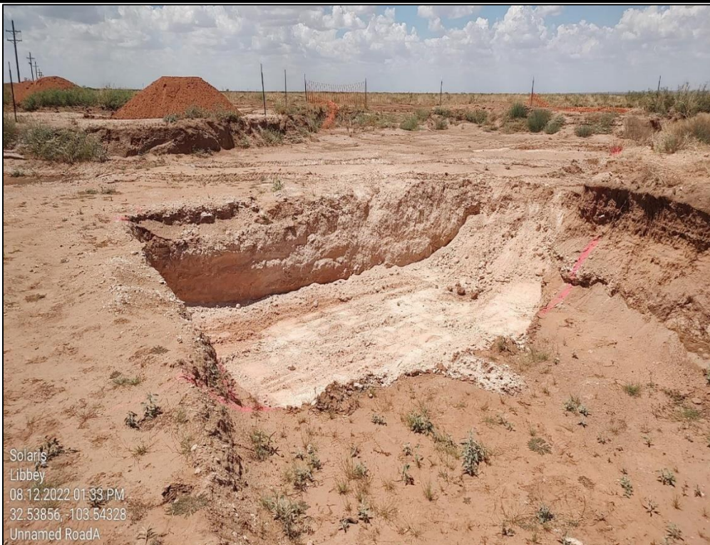
PHOTO 17: View of excavation area CS39
