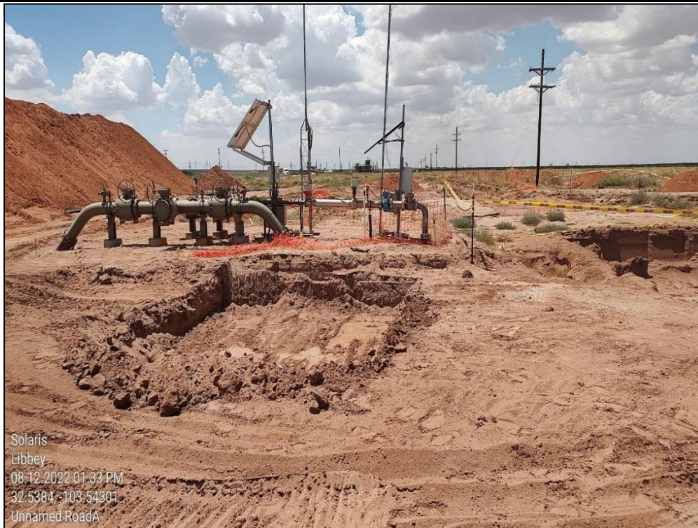
PHOTO 16: View of excavation area CS33
