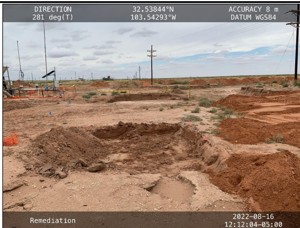
PHOTO 20: View of backfilling of excavation
