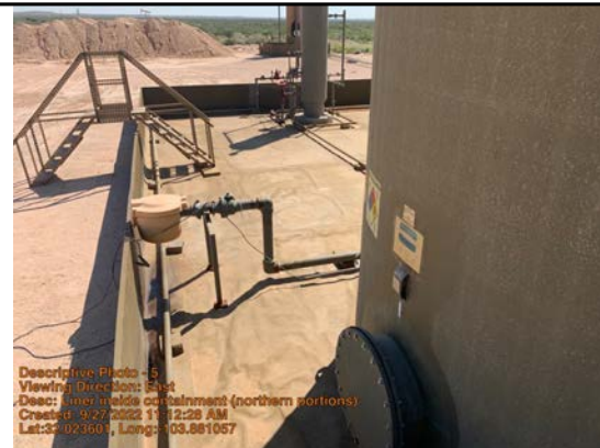
Liner inside containment (northern portions)
