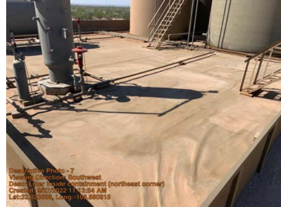
Liner inside containment (northeast corner)
