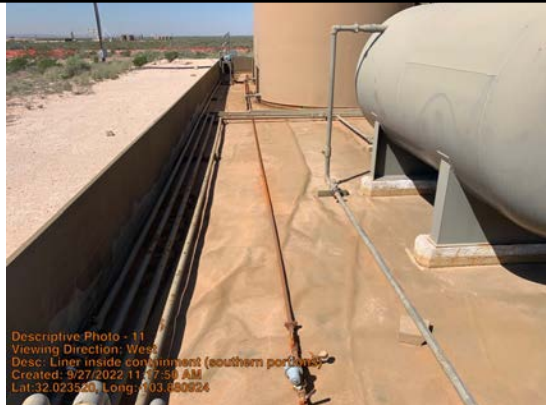
Liner inside containment (southern portions)
