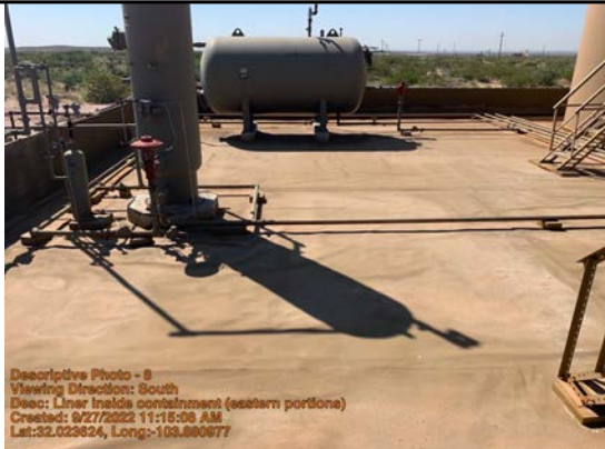
Liner inside containment (eastern portions)
