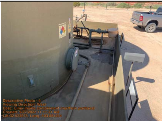
Liner inside containment (northern portions)
