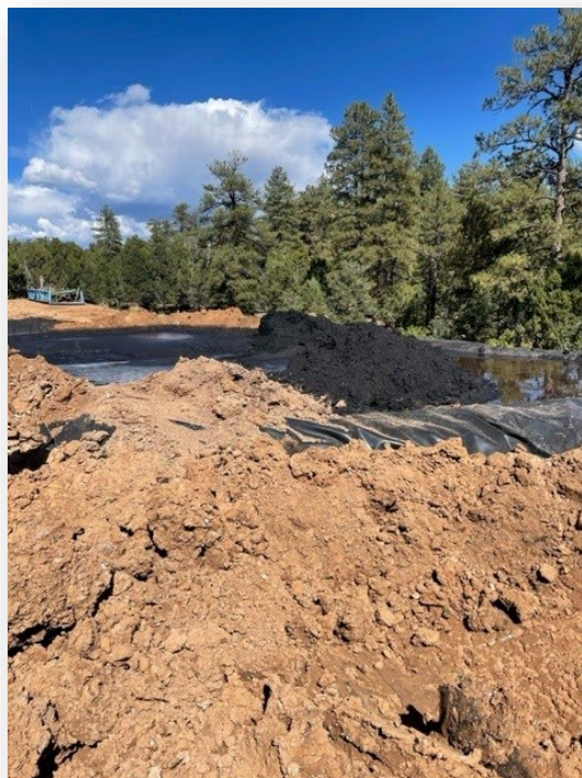
Figure 1. Pit with Produced Water and Coal Cuttings
