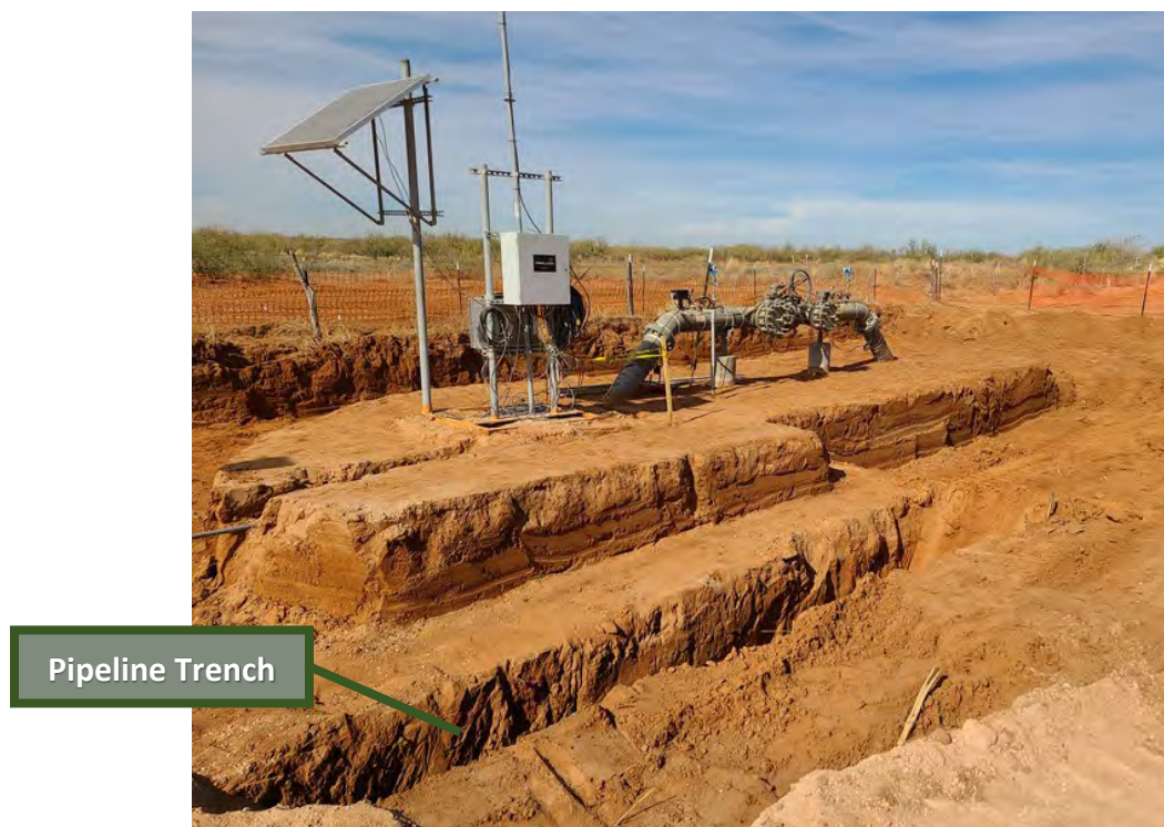
Figure 3: Excavation around pipeline riser, solar panel, and supporting utilities. Photo is viewing northwest. 11/22/2022. 32.0375283, -103.2785425.
